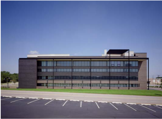
South elevation from the parking lot across the street.
