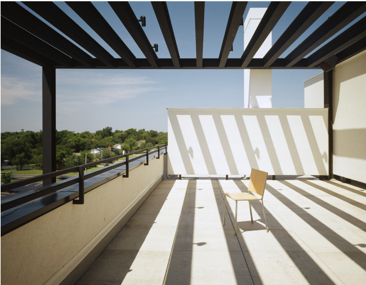
Roof deck and trellis.
