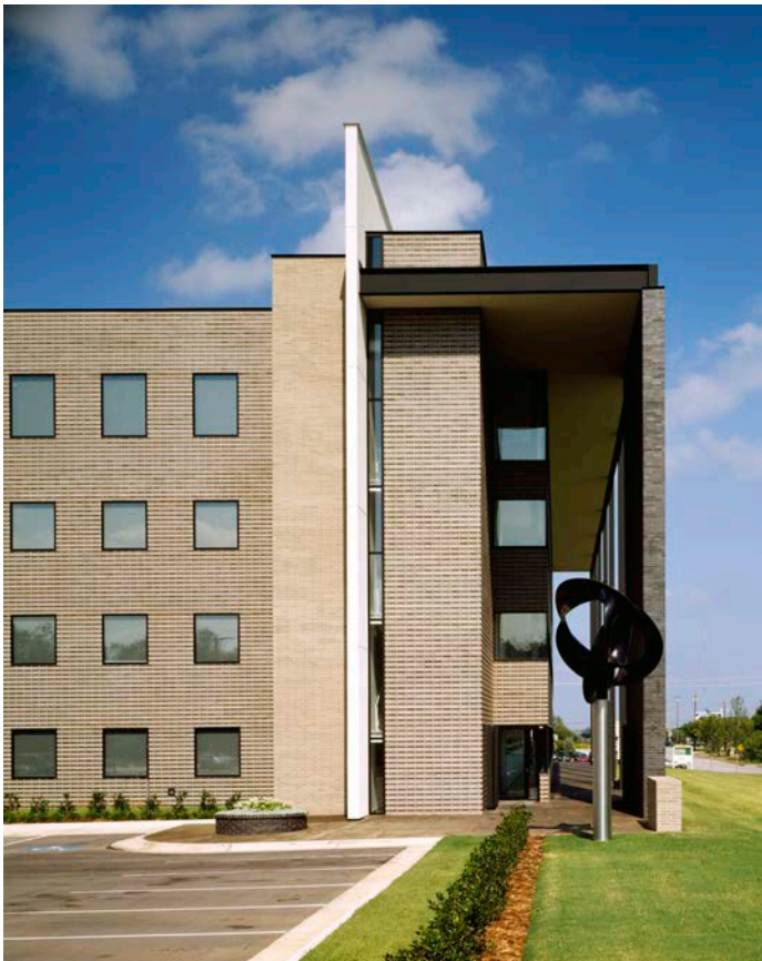
West elevation at Main entry. The punched windows respond to the adjacent residential neighborhood to the west.
