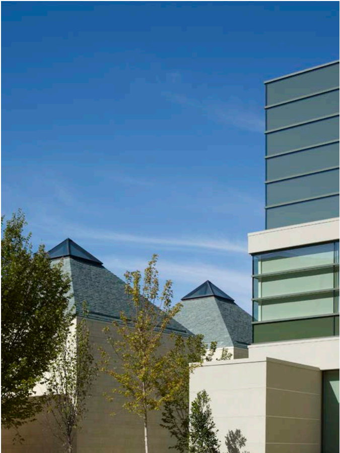
Southwest corner detail of Stuart Wing.
