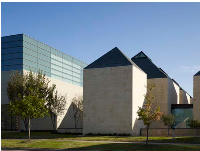
Detail of northwest corner of Stuart Wing. Building with pyramid roofs is existing Lester Wing.
