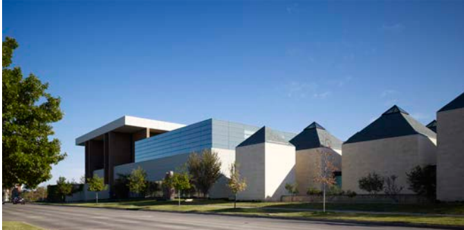
Exterior view looking southeast.
