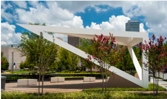
A detail view of the pavilion structure. The concrete buttress allows the cantilever.
