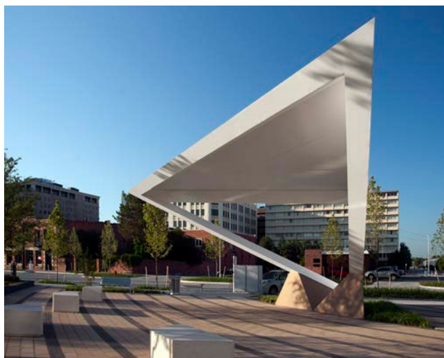
A detail view of the pavilion structure. The concrete buttress allows the cantilever.
