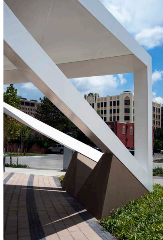
A detail view of the pavilion structural corner and the concrete buttress.
