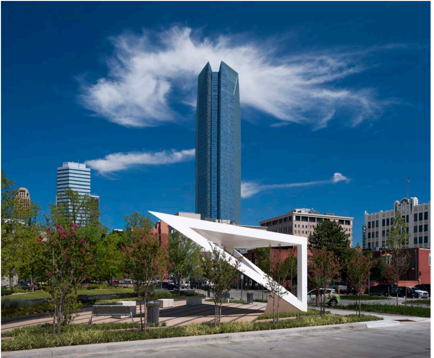
The sculptural pavilion makes a clear statement about 21st Century forms and the connection to the park's history. Old and new live together in harmony. We are a progressive city with a rich history.
