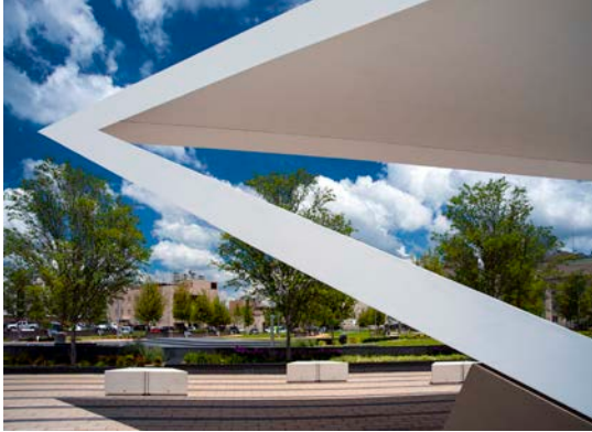
A detail view of the sharp edged, triangular shaped structural members of the pavilion framework.
