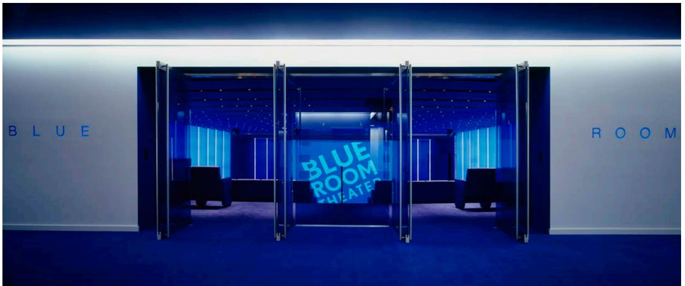
Looking north at glass entry doors. Both entry doors and glass sidelites are blue laminated glass.
