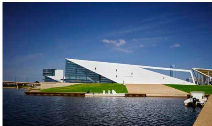
The east elevation is parallel to a river inlet allowing rowing shells to access the river via a concrete ramp. The inlet size allows for a 60' long boat to maneuver. The open beam frames Downtown. The gold "notes" are rhythmically placed on the façade.
