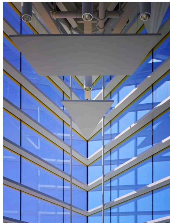
Performance Hall detail of building “nose.” Ceiling panels provide acoustical tuning and obscure acoustical surfaces.
