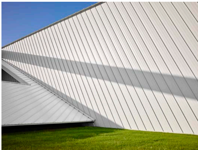
The northeast corner of the building is defined by the picture frame wall and an early morning shadow. The mechanical enclosure on the left provides sculptural protection for systems. It is also one of the best places to backdrop a concert.
