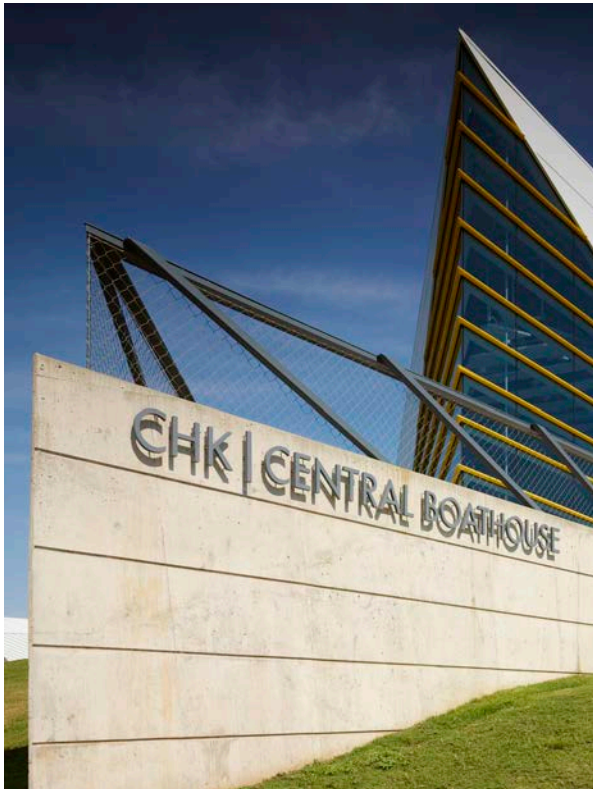
The concrete prow provides an elevated view of the river and acts as a barrier for occasional flooding.
