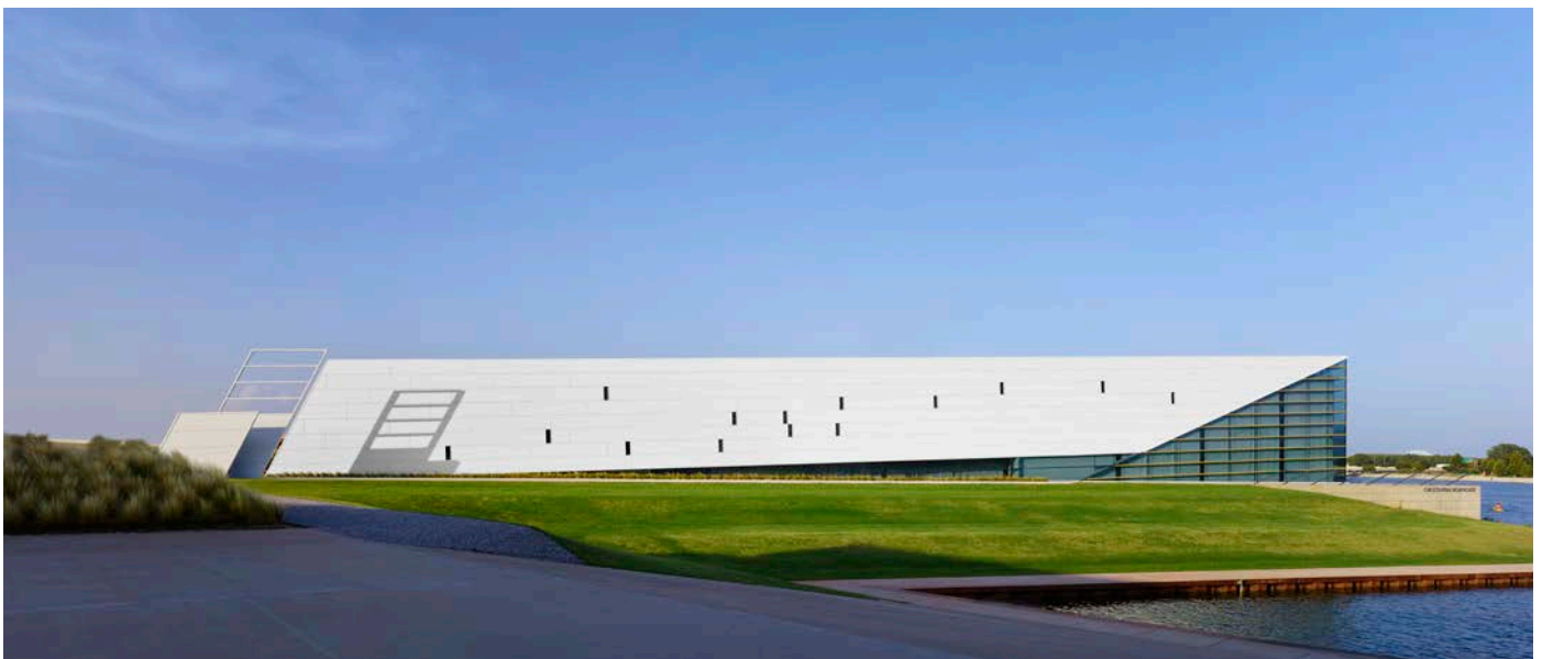
The west elevation illustrates the gold glass “notes” and the connection between rowing, fine art, and music. Simply summarized as rhythm .
