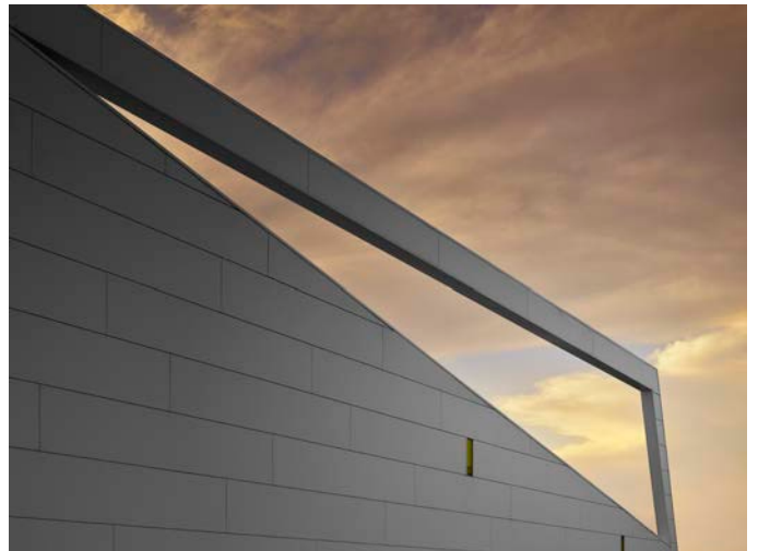
The northeast wall opening frames last minute views of sunset.
