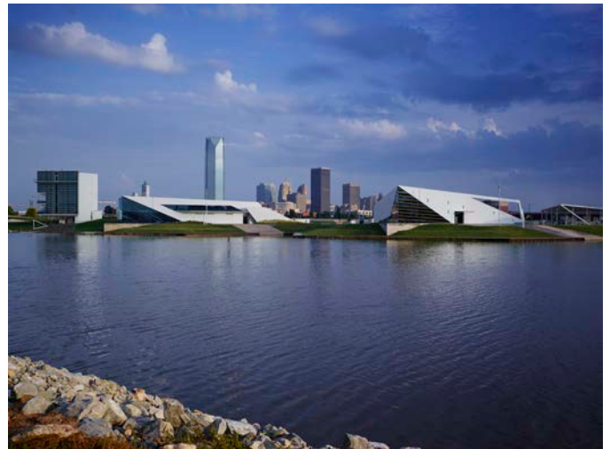
The boathouse “floats” in the water. The Boathouse District has become a great place for family entertainment & healthy play.
