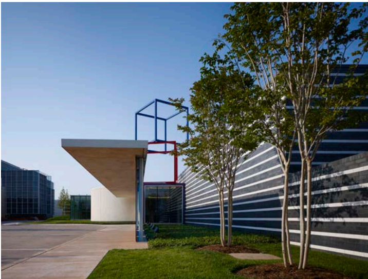
Main entry detail of canopy.
