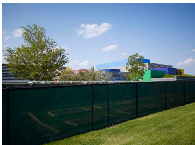
North elevation behind construction fence and temporary children's vegetable garden in the foreground.
