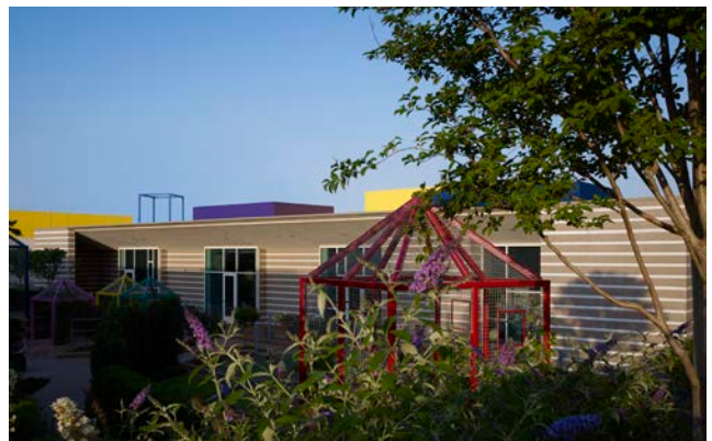
West elevation of north courtyard looking southwest.
