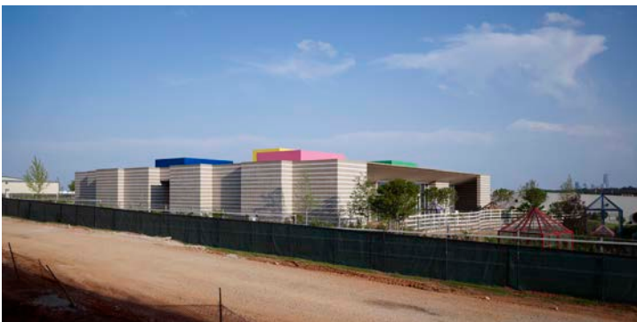
North elevation of east section with courtyard on right. Notice colored mechanical enclosures on roof.
