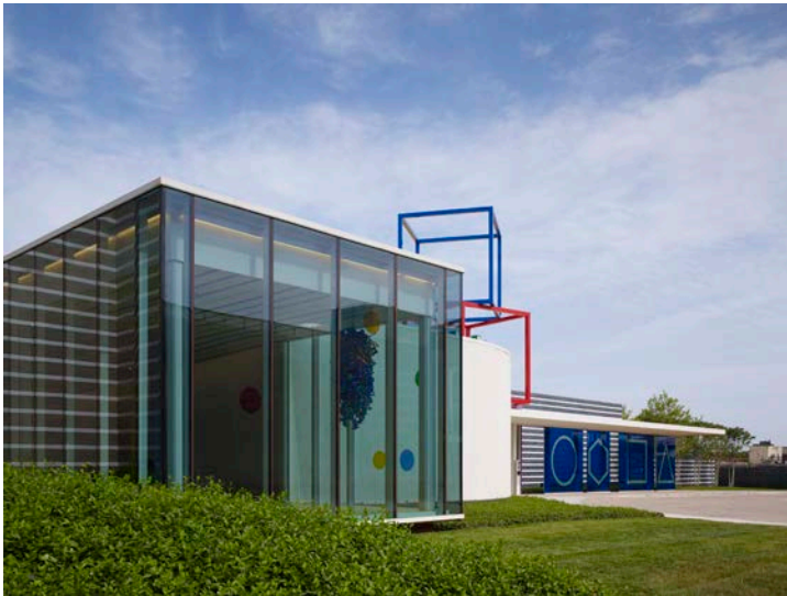
West elevation main entry with glass ramp enclosure.
