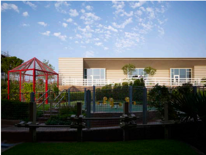
West elevation inside north courtyard looking east.
