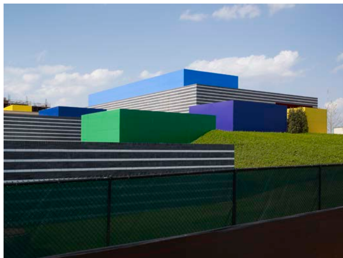
Detail of south elevation/east section showing colored mechanical enclosures.
