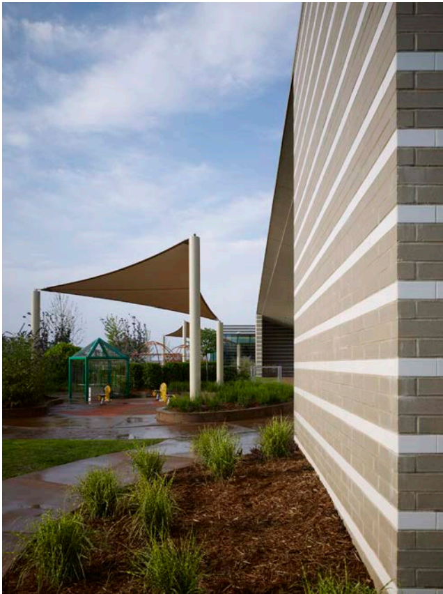
East elevation and east playground looking south.
