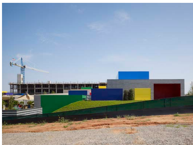
North elevation of east section from adjacent construction site.
