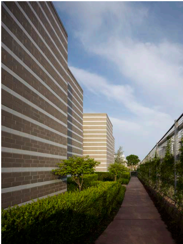
North elevation walkway looking west.
