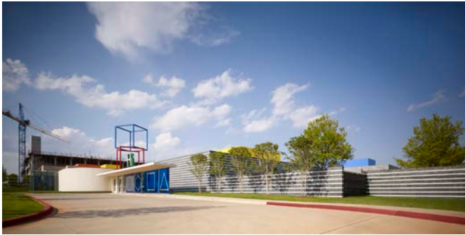
West elevation looking northeast.
