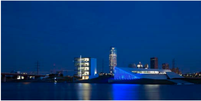
Dusk View looking northwest at Chesapeake Finish Line Tower and the Devon Boathouse
