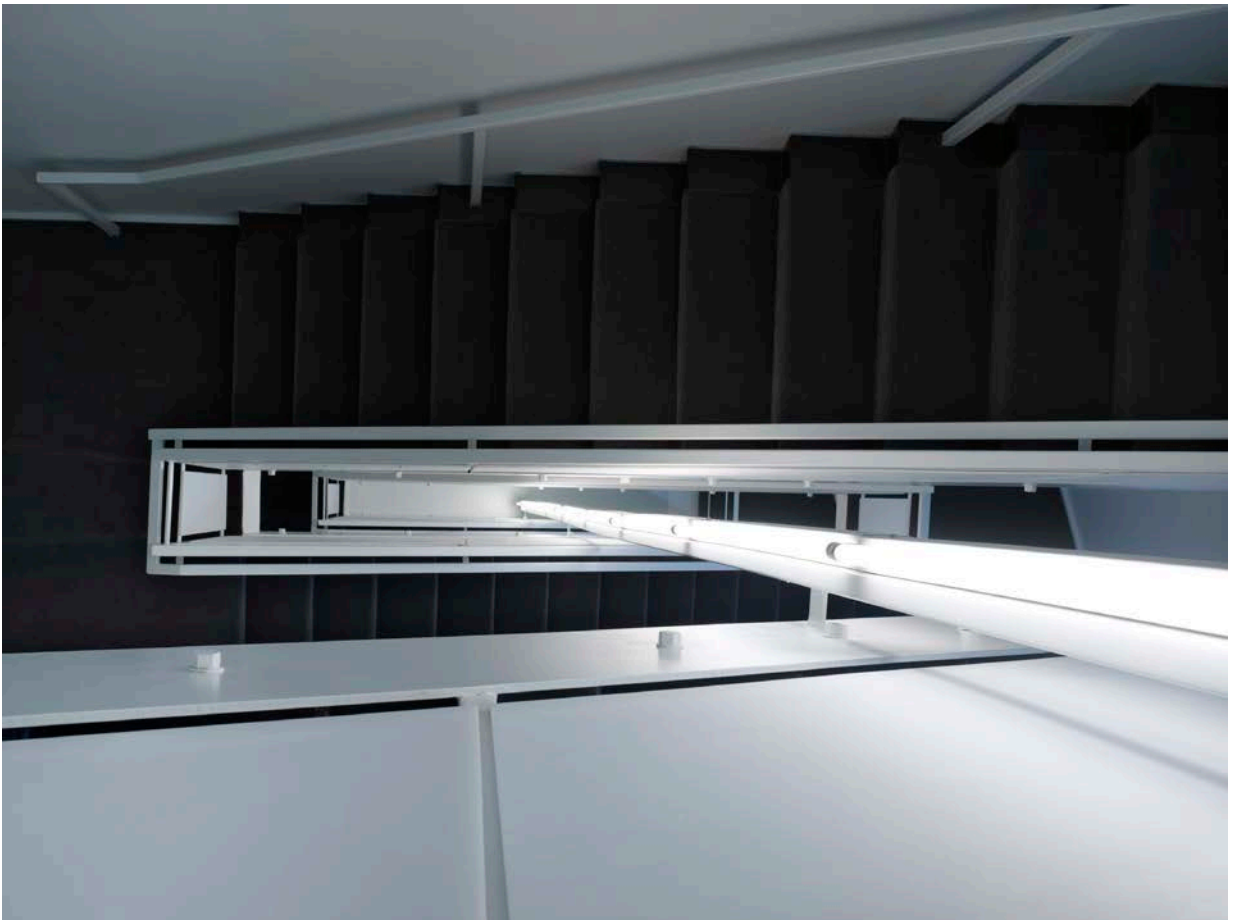
Overhead view of stair lighting detail
