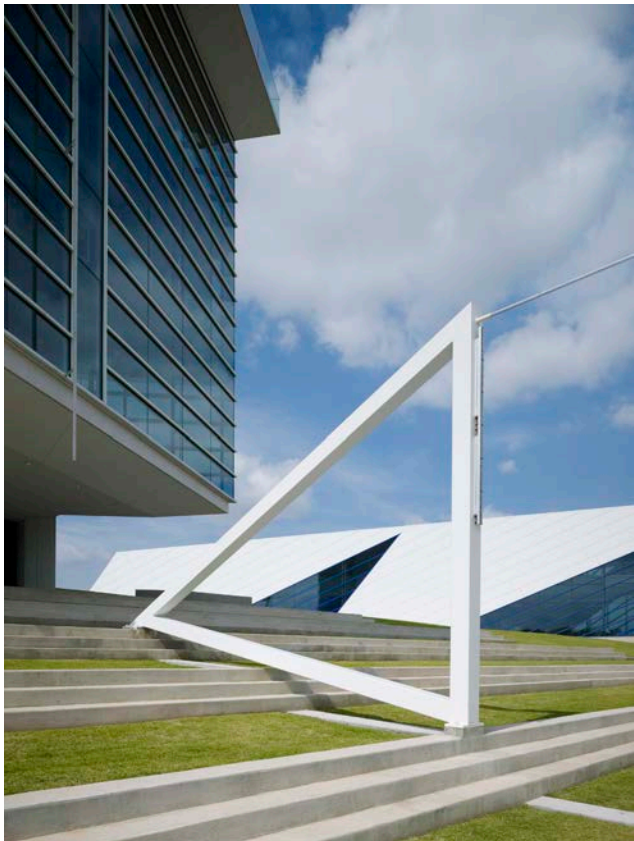
Southeast elevation detail and finish line cable structure
