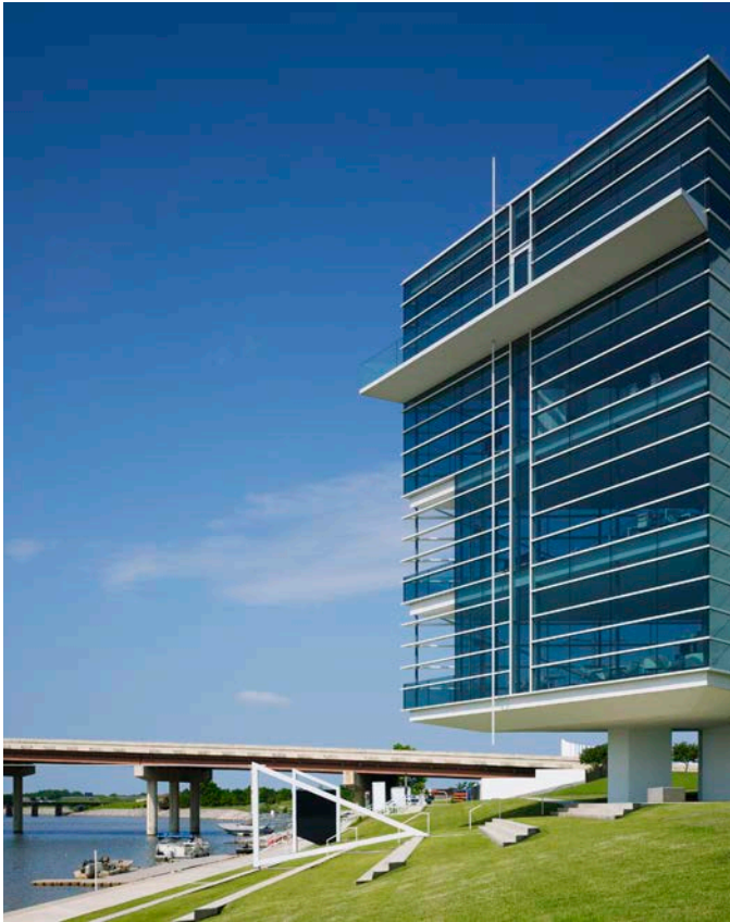
Southeast elevation showing balconies
