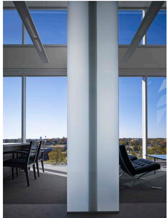
Laminated glass detail between reception area and executive office. Clerestory window is exposed.
