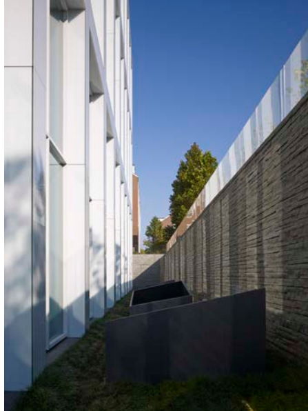
Atrium view looking north on east side.
