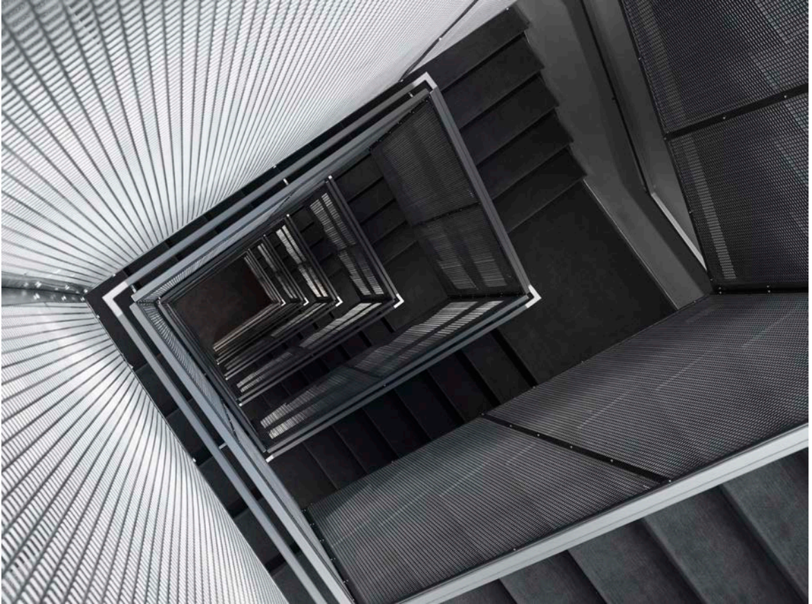
Detail of interior stair showing square perforated aluminum panels.
