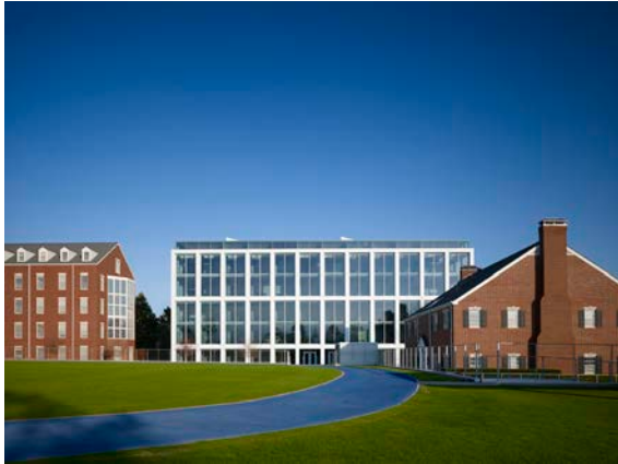
West Elevation at midday. The window proportion of the red brick buildings is consistent with the Building One.
