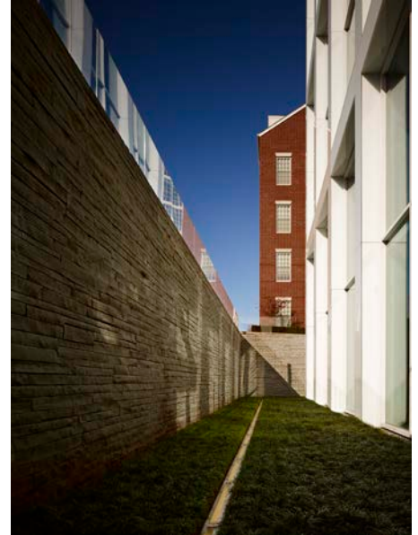
Atrium view looking north from west side.
