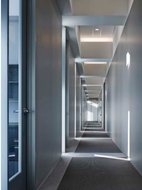
Corridor view looking north with glass doors and slit windows allowing light from the perimeter to the interior.
