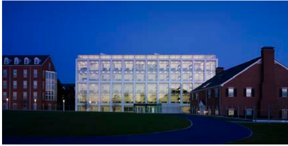
West Elevation at sunset. The window proportion of the red brick buildings is consistent with the Building One.
