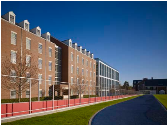
Building One is adjacent to the Central Park Parking Structure and the soccer field.
