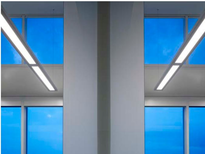
Fifth floor clerestory detail with etched glass endcap and suspended lights.
