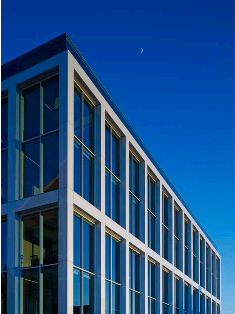
Southeast building corner illustrating white glass rain screen, the fourth clerestory. White gaskets make the glass openings crisp.
