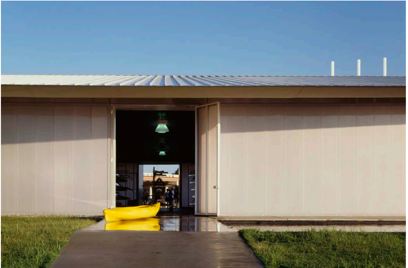
North elevation boat storage access door
