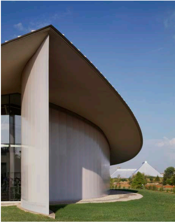
Northeast rooftop and "rudder"
