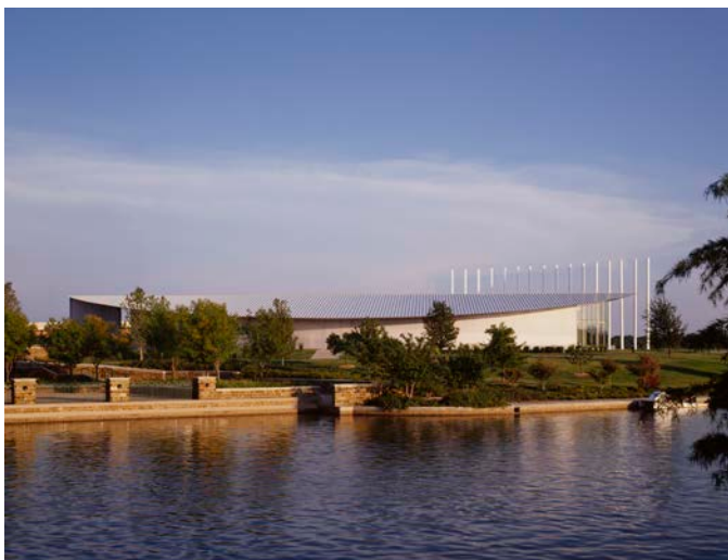
Northwest elevation looking southeast
