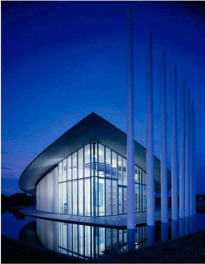
Southwest corner showing entry, deck, reflecting pool and steel pylons
