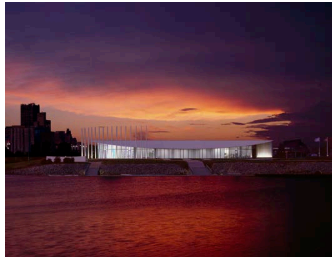
South roof cantilever looking east
