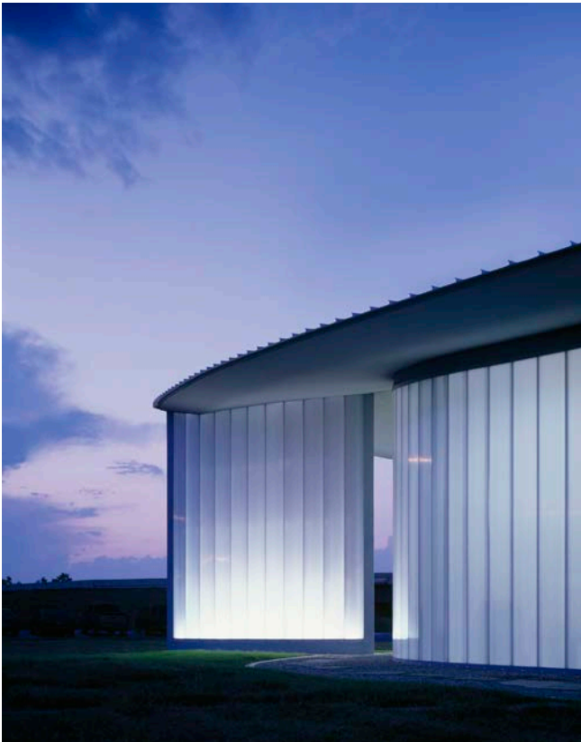
Northeast corner looking east towards the "rudder"
