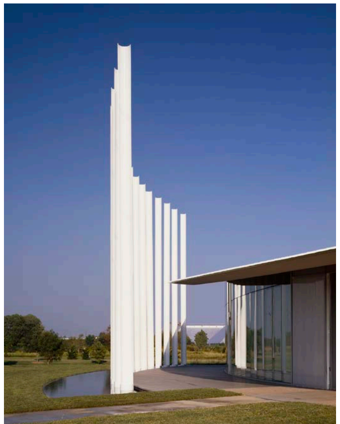
South elevation looking west
