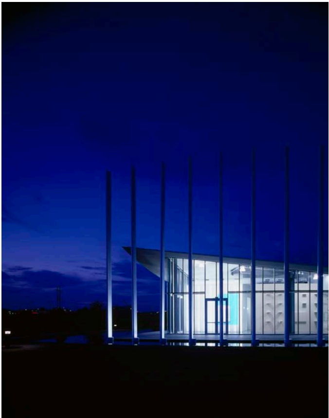
South elevation looking north
