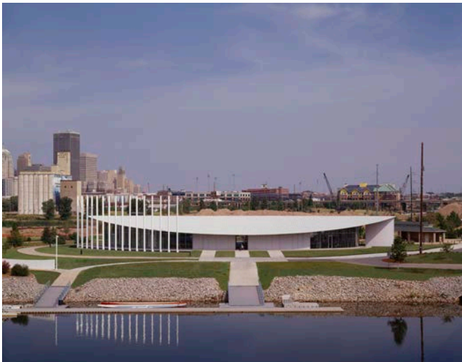
Southwest corner looking north
