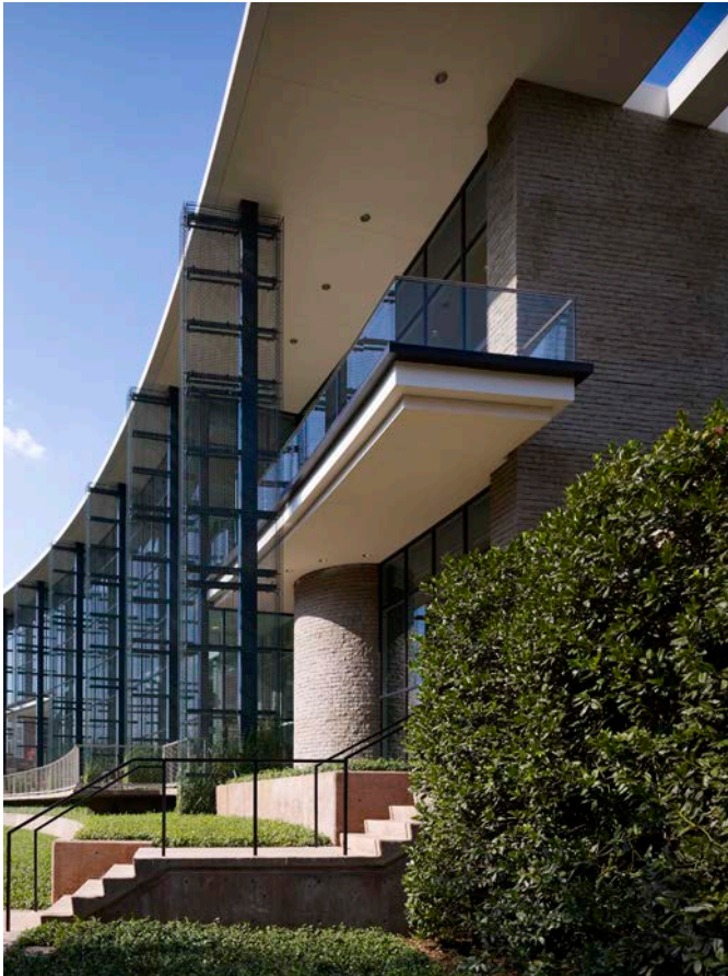
West elevation/detail of 2nd floor balcony. Notice green screen clad columns for Coloratus.
