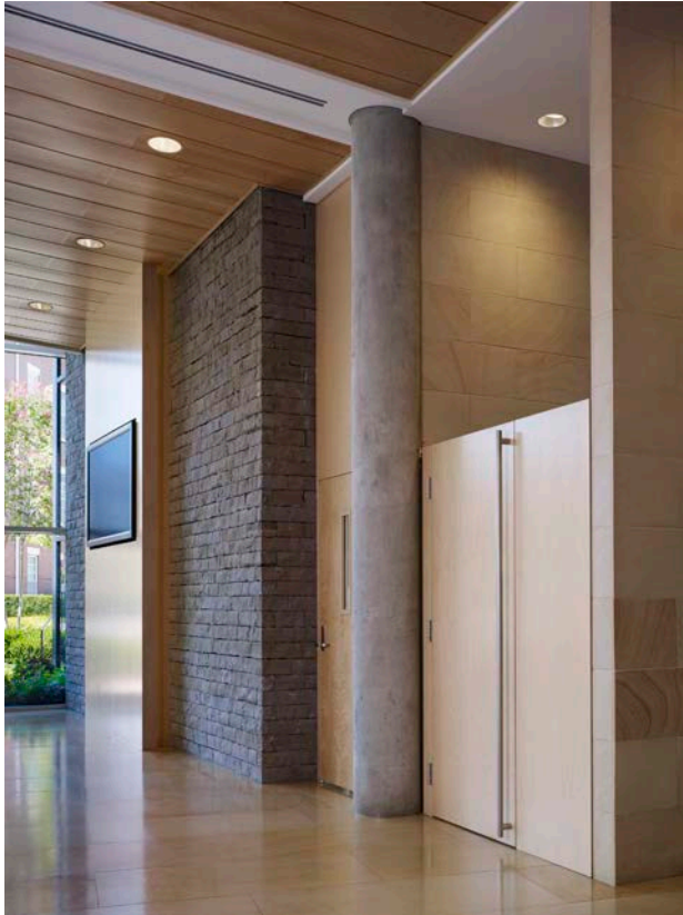
East wall of the main dining room with exposed concrete column, limestone walls and wood doors.
