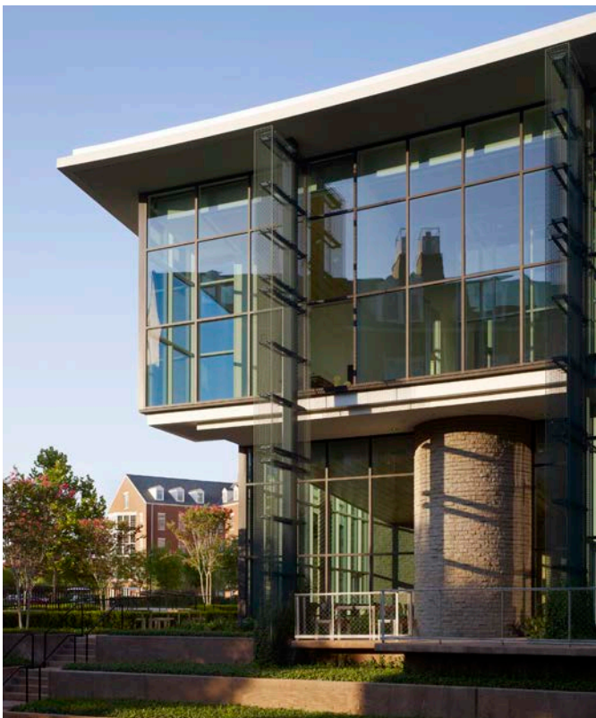
Northwest corner detail with cantilevered corner and stone cylinder
