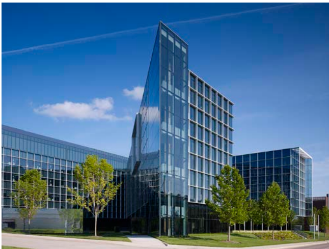
View looking southeast at the stair wing for Building 14. The square grid Brise Soleil was created to connect the architecture to the precision of the IT department.
