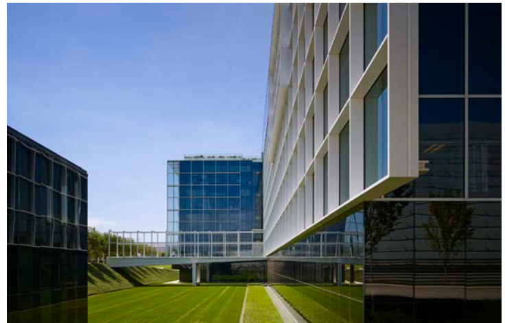
The northeast corner looking south. The site drops 10 ft. to create a pocket park. On the roof of the east/west wing is the outdoor dining space.
