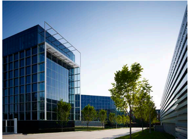
A view looking west southwest at the north elevation of the office space with Skyline Restaurant on the top level. The glass portal provides west sun protection. The open frame is an LED light.
