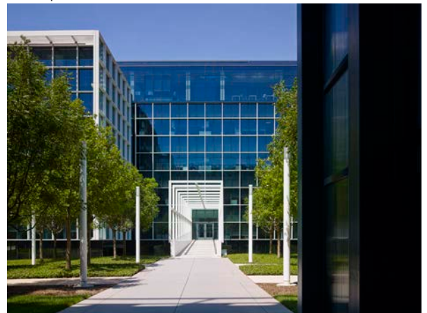
A view looking west from Car Park Three towards the main entrance which is a bridge enclosed by a tubular portal. Skyline restaurant on the top floor is articulated differently than the main building skin.
