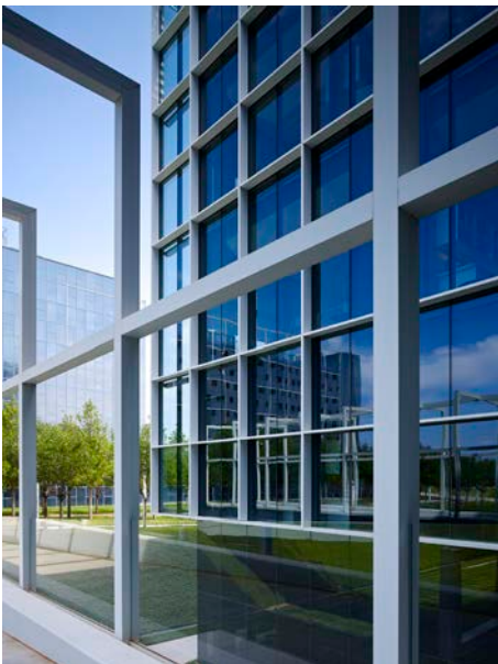
A detail of the entry bridge on the east side of the building. The square grid translates to become structure for the bridge entry.
