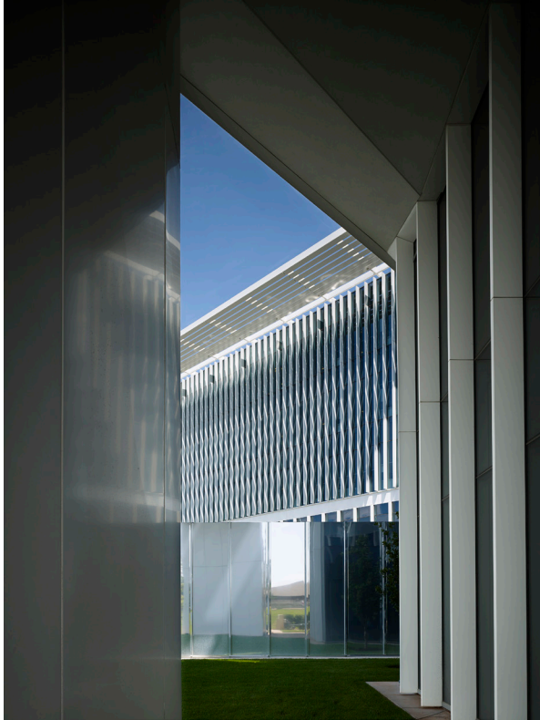
A view through the corner portal frames the shadows.
