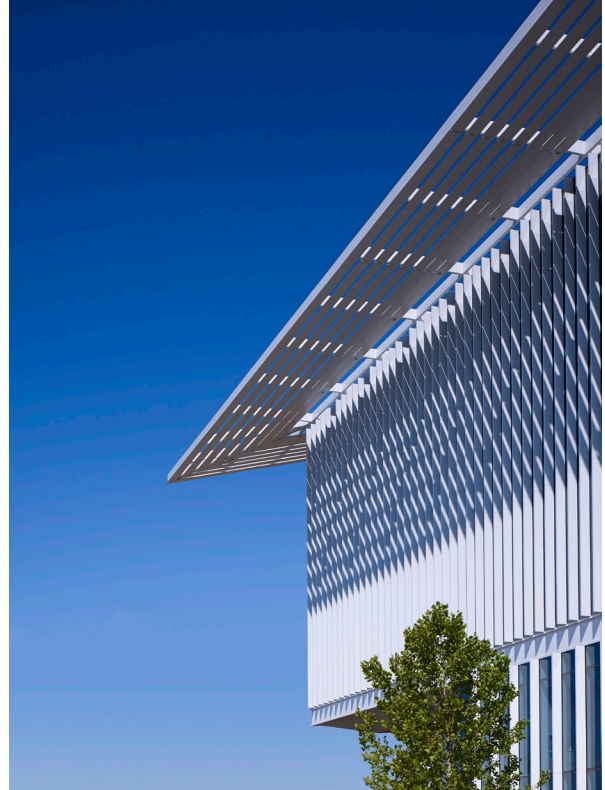
The southwest corner/elevation illustrates the effectiveness of the roof edge sunscreen. In the middle of summer the entire south façade is in shade.
