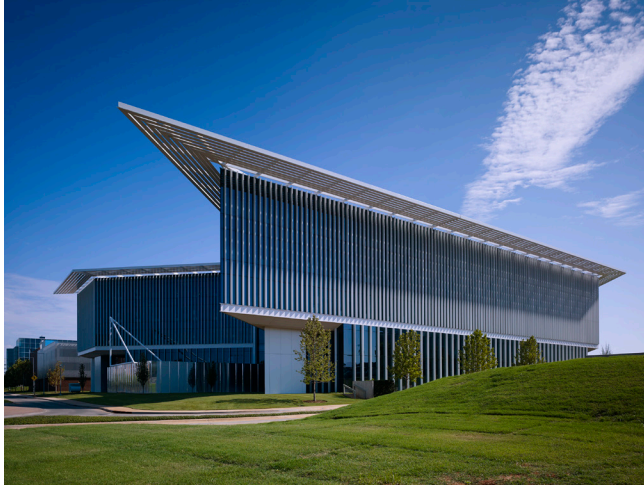
The southwest corner of the campus entry, Building 15 stands as landmark building representative of the corporate dynamics.
