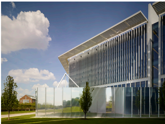
The west elevation illustrates the roof edge sunscreen, glazing vertical fins and the polished stainless steel mechanical enclosure.
