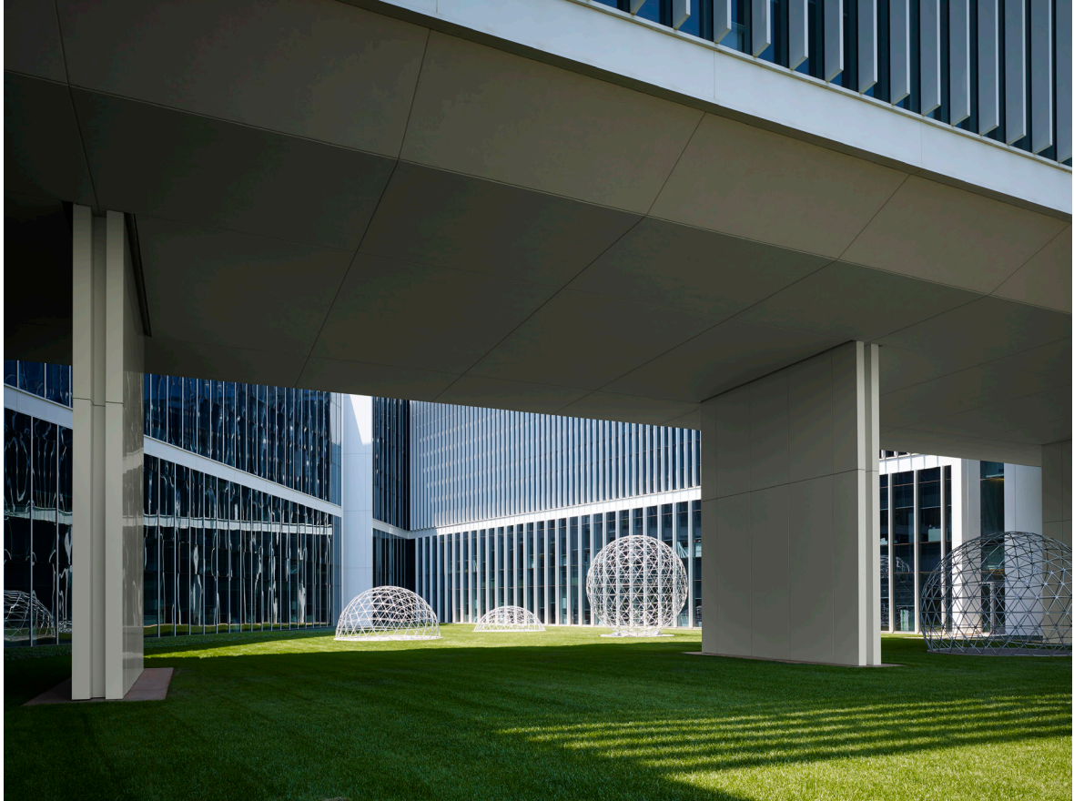
A view under the east building bridge defines the courtyard.
