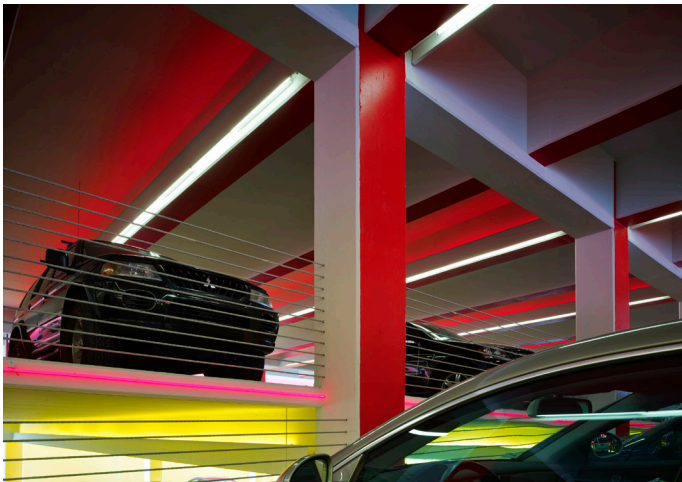
The cast in place concrete structure, tension cable rails, and color combine to create a memorable statement about parking.
