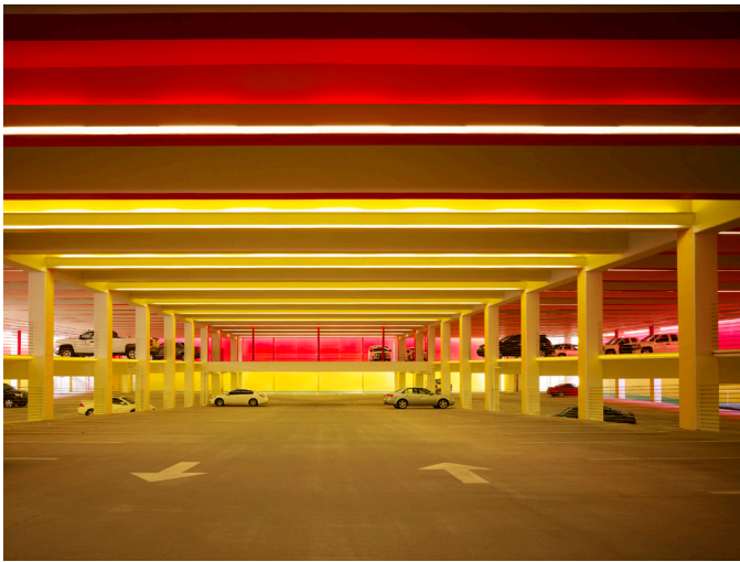
The main entrance is a surprise because you enter into a two-story central ramp and the color wayfinding system begins to unfold. The entire perimeter is an open atrium and allows sunlight to move in and out of the space. The changing shadows animate the room.
