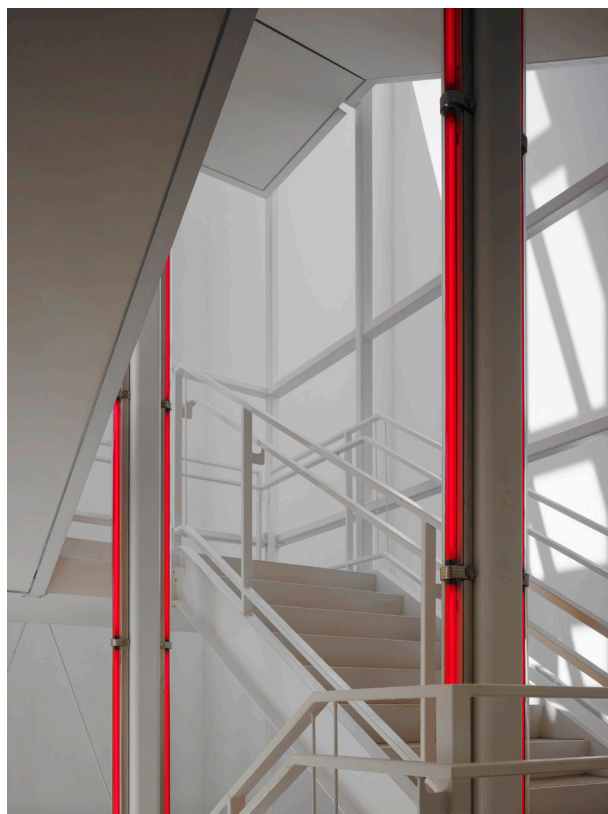
A detail of the red stair showing the vertical colored lighting fixtures and a sliver of daylight coming in along the edge.
