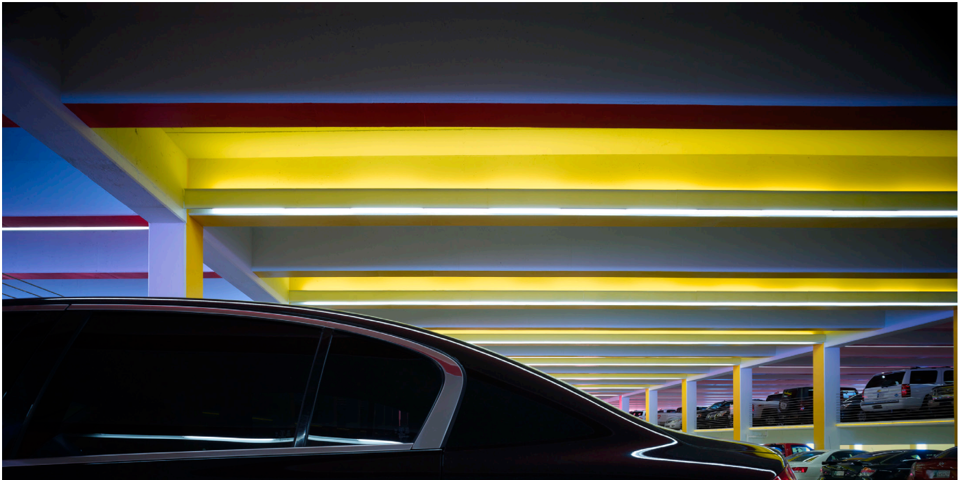
The central ramp open volume changes your perspective about parking structures. Unlike other structures, your ability to understand location, your appreciation for safety, and the color combine to make the parking experience fresh and new each time you visit.
