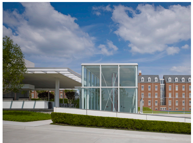
Northwest corner stair tower adjacent to the North Pavilion and surrounded by existing campus buildings. The colored light allows each stair tower to be a part of the wayfinding system.
