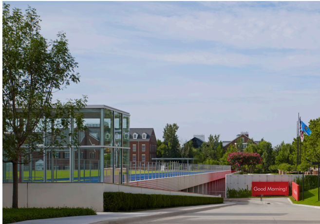
Looking south at the west entrance into the Central Park structure. Glass stair towers anchor the corners, and a soccer field/running track create a central green space in the campus. Our client loves a morning and evening greeting as a way of engaging employees.
