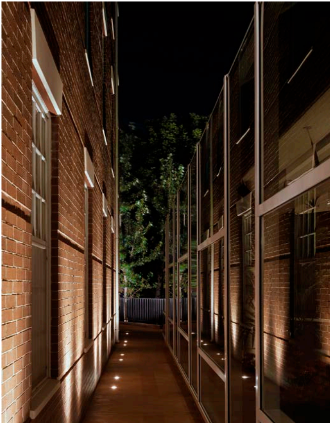
View looking south at walkway between existing brick building area near glass structure.
