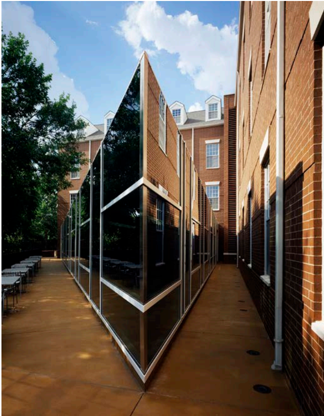
View looking north from knife edge with walkways on both sides.
