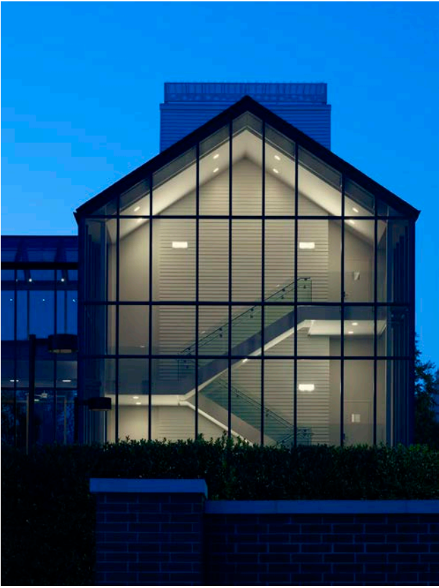
South elevation of east addition.
