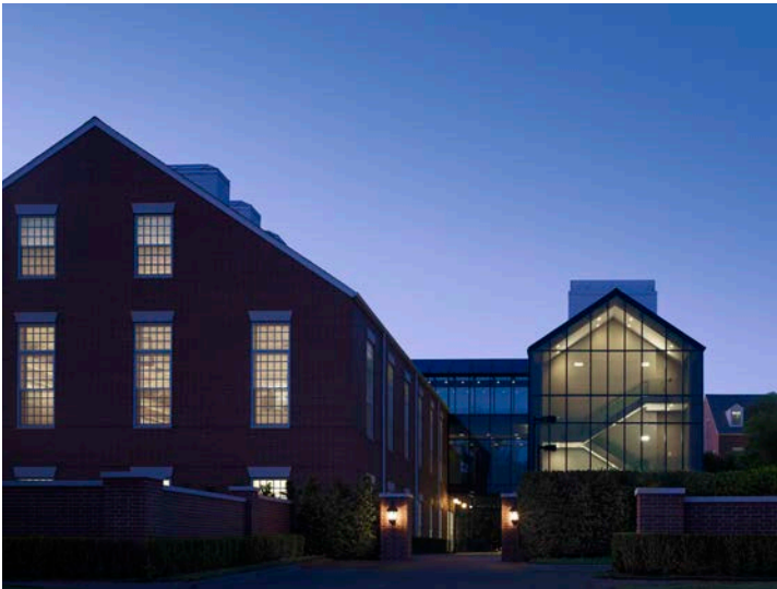
Dusk view of new addition with existing building on the left.
