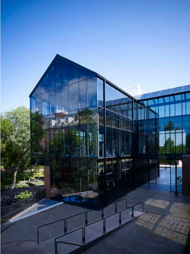
View from existing building window to east addition.
