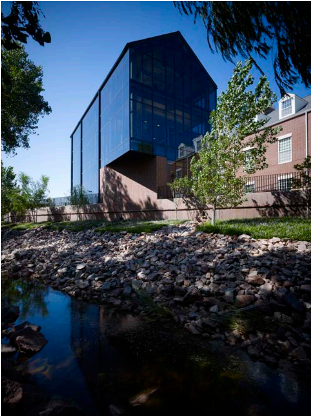
Northeast corner from existing natural creek.
