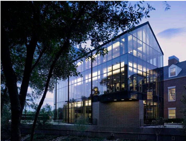
View from northeast looking southwest.
