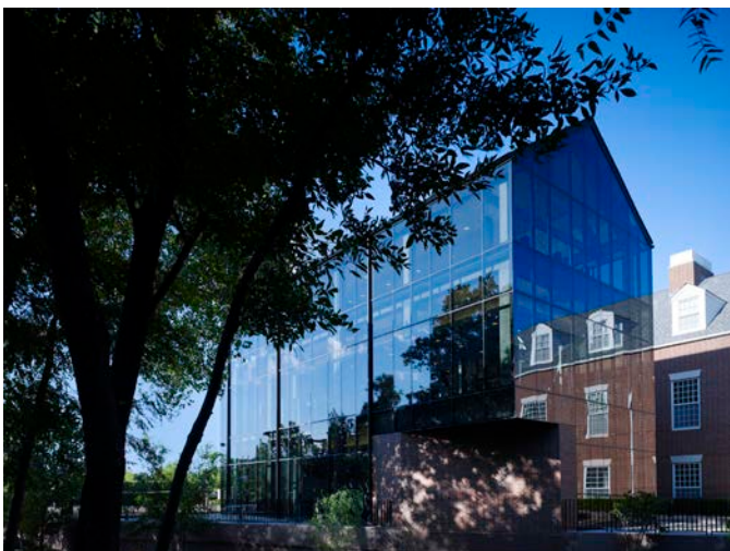
Northeast corner from existing natural creek.
