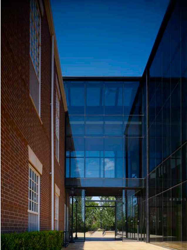
South entry breezeway connection.
