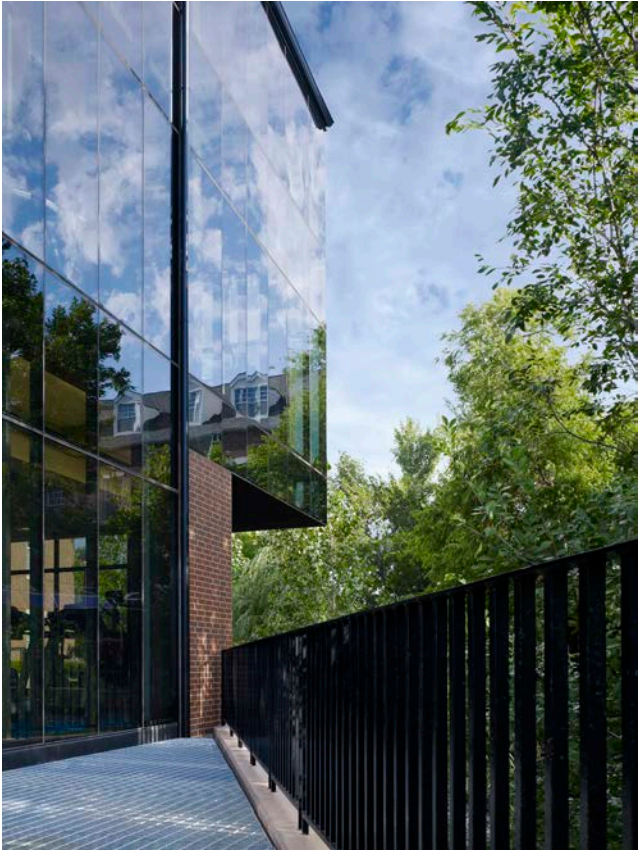
Northeast corner detail
