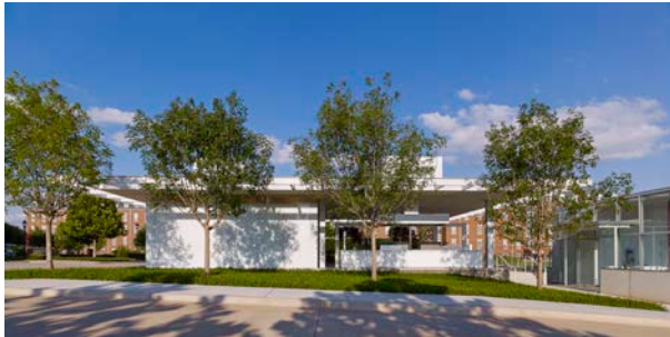
West elevation showing the white glass skin, clerestory windows, food service counter and parking structure stair enclosure on the right. In the foreground is the entry drive for the parking garage.
