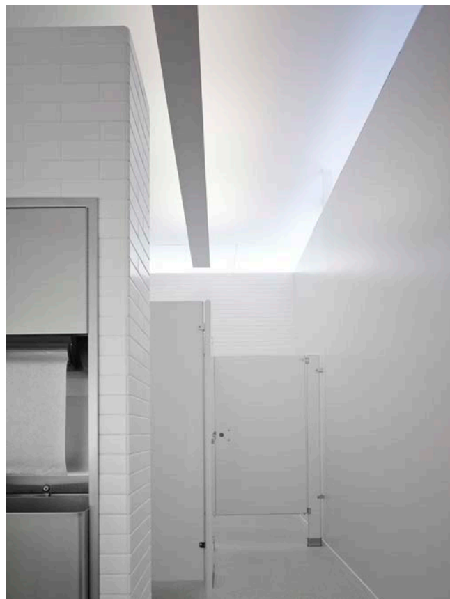
Men's toilet looking west illustrating the attention to detail, clerestory lighting and indirect lighting. The floor is white terrazzo. The walls are white tile.
