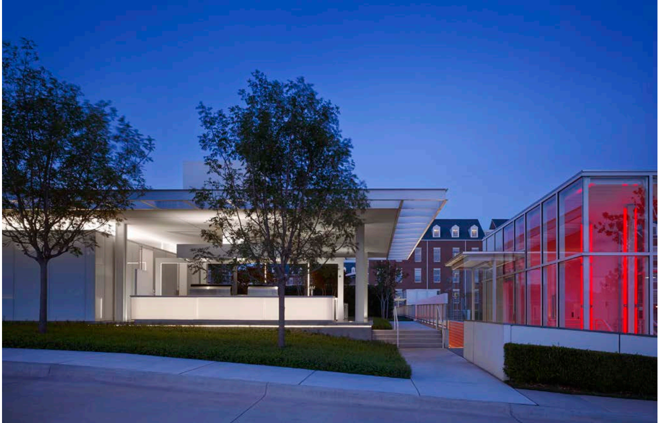
Partial view of the pavilion and the parking structure stair tower looking east at dusk. The colored lighting in the stair tower acts as wayfinding.
