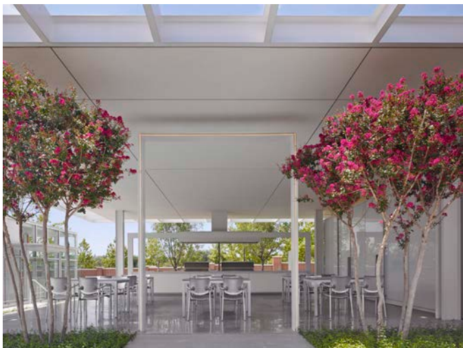
LED portal entry onto the pavilion deck crossing a perforated steel ramp. Toilet facilities are housed in the space to the right, and food preparation is provided with the open kitchen.
