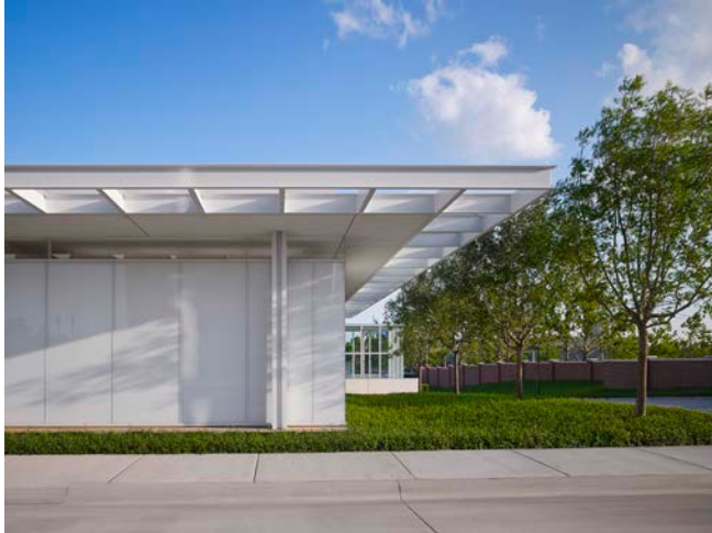
Northwest corner of the structure showing white glass skin, clerestory windows, exposed steel columns and sunshade roof. The parking structure stair enclosure is beyond
