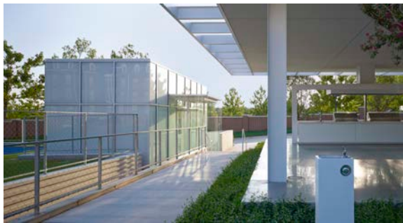
View from the east looking west under the pavilion roof with the parking structure stair enclosure on the left.
