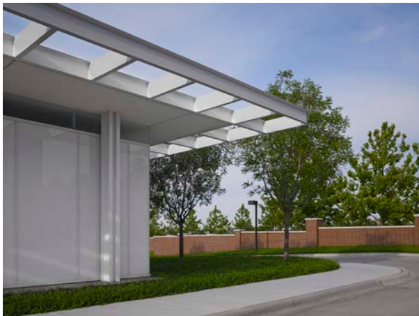
View from the north looking southwest showing the clerestory window, freestanding column and Brise Soleil.
