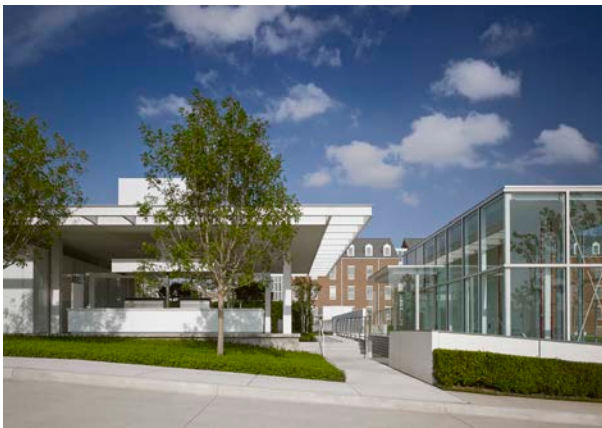
Partial west elevation showing the open perimeter roof edge, food service area, and parking structure stair tower.
