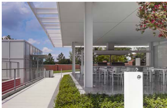
The water fountain is given as much attention as the steel detailing of the pavilion. The building slab is polished concrete and floats above the landscape surface.
