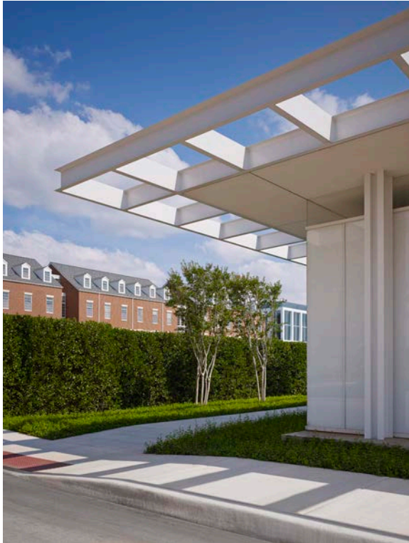
Northeast corner looking southeast showing clerestory glass freestanding column and Brise Soleil. This view puts the pavilion project in context with the existing campus.
