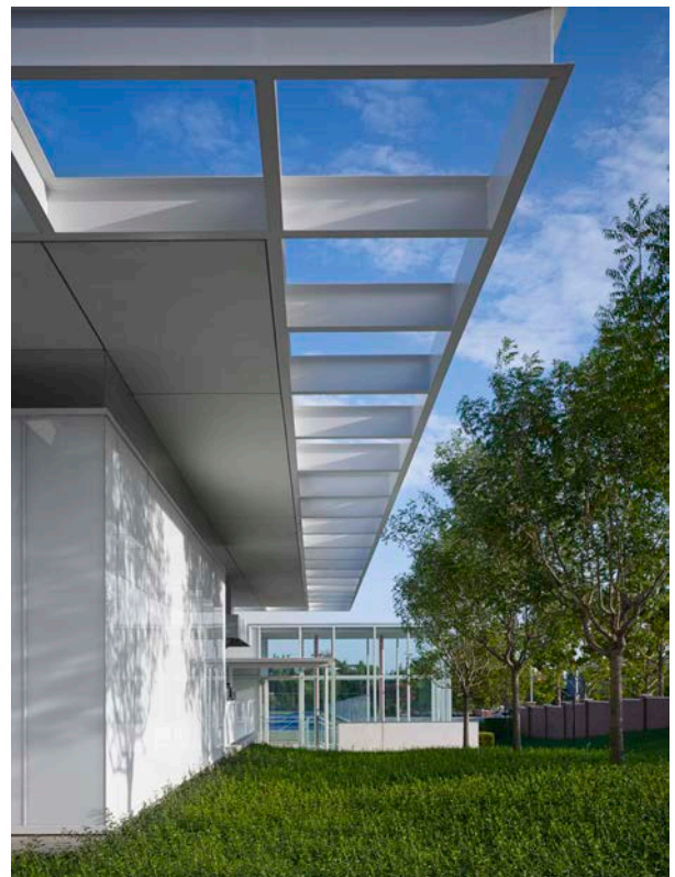
The northwest corner detail looking south with white glass skin, clerestory windows and sun shade roof. The parking structure stair tower is visible beyond.
