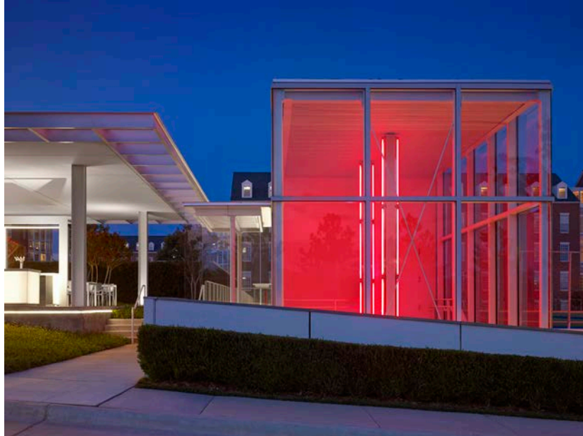
Detail view of the pavilion and the parking structure stair tower looking east at dusk. The colored lighting in the stair tower acts as wayfinding.
