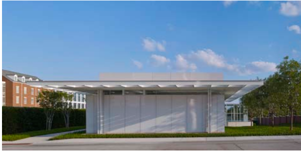
North elevation showing white glass skin, exposed columns, extended roof and sun shade perimeter
