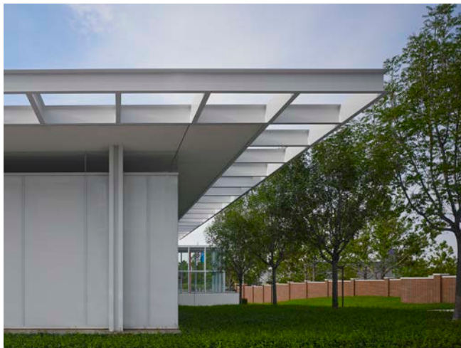
View from the north looking south showing the clerestory window, freestanding column and Brise Soleil.
