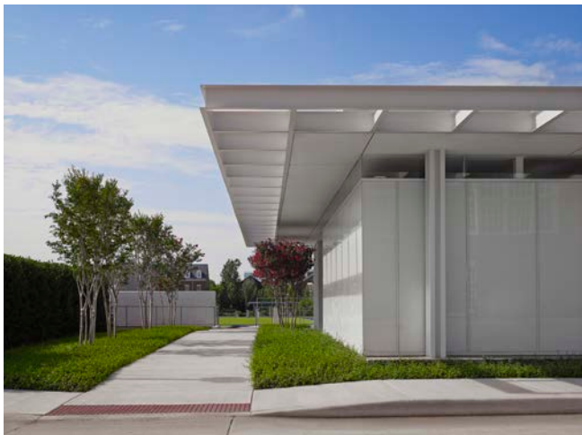
View from the northeast corner looking south showing the clerestory window, freestanding column and Brise Soleil.
