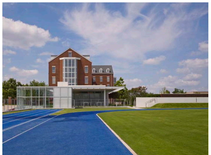
View looking north from sports field toward the pavilion and the parking structure stair enclosure. On the right is an earthen stage used for events. Below the sports field surface is a 2 1/2 story parking structure. The North Pavilion is used for warm-up, toilets, and refreshments.
