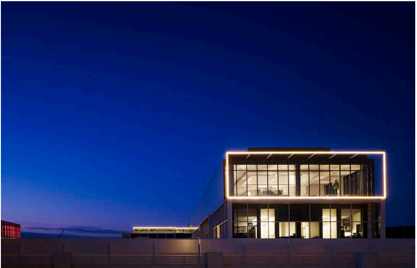
The north elevation of the 6th floor restaurant with the signature LED light line.
