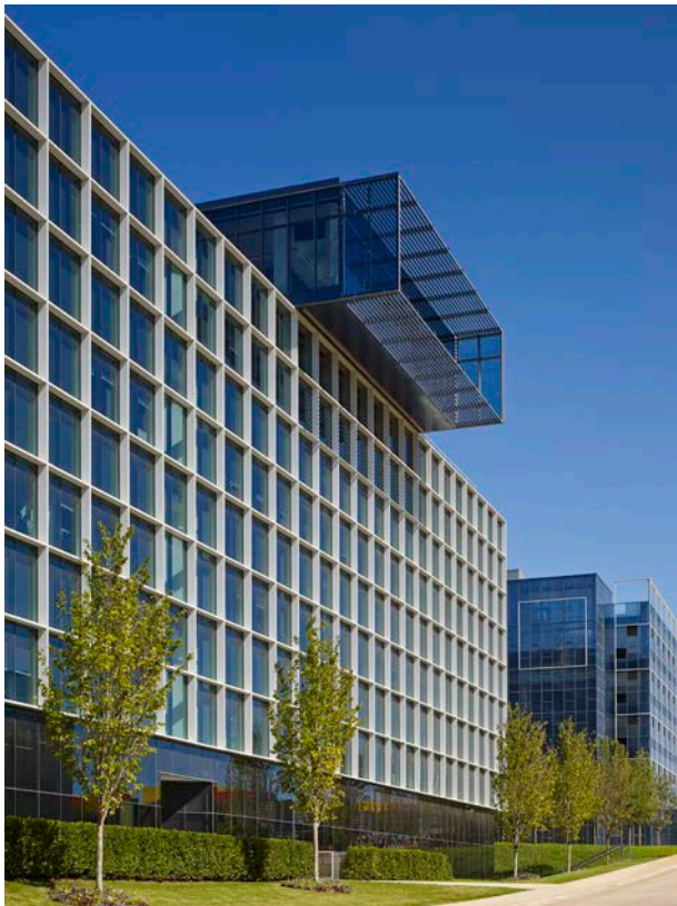
The south elevation of Chesapeake Building 14 with the 6th floor Skyline Restaurant cantilevered over the edge. The form frames the downtown view. The lattice creates sun shading. An LED light line defines the architectural form and provides intrigue from afar.
