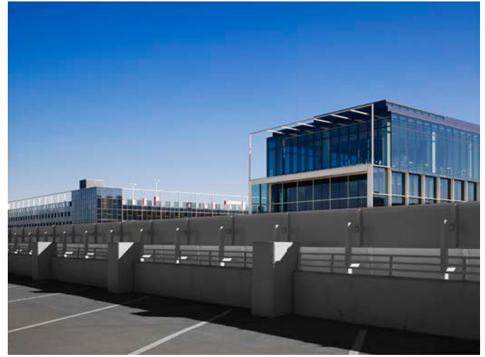
A view looking southeast showing the north end of the Skyline Restaurant from the Parking Structure 1 on the north. Parking Structure 3 is beyond and on the left.
