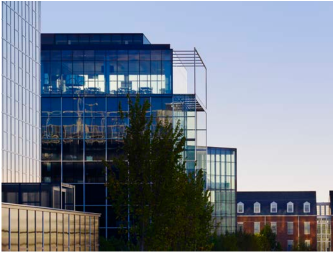
A view showing the northeast elevation and the 6th floor frame extension. The LED light line is visible on both ends of the restaurant form.
