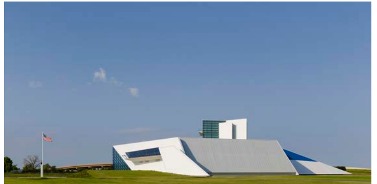
View looking Southwest showing east balcony
