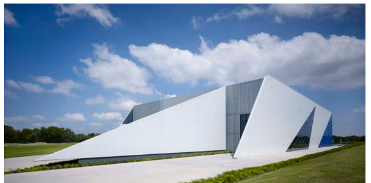
Northwest corner of the building at main entry
