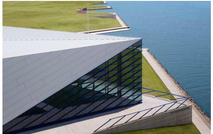
Partial west elevation and roof. Notice there are no exposed mechanical devices on the roof
