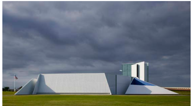
North elevation with Chesapeake Finish Line Tower in the background. The mechanical enclosure is on the right.
