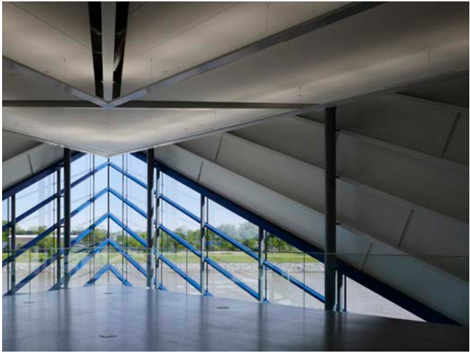
2 nd floor viewing room looking south toward river
