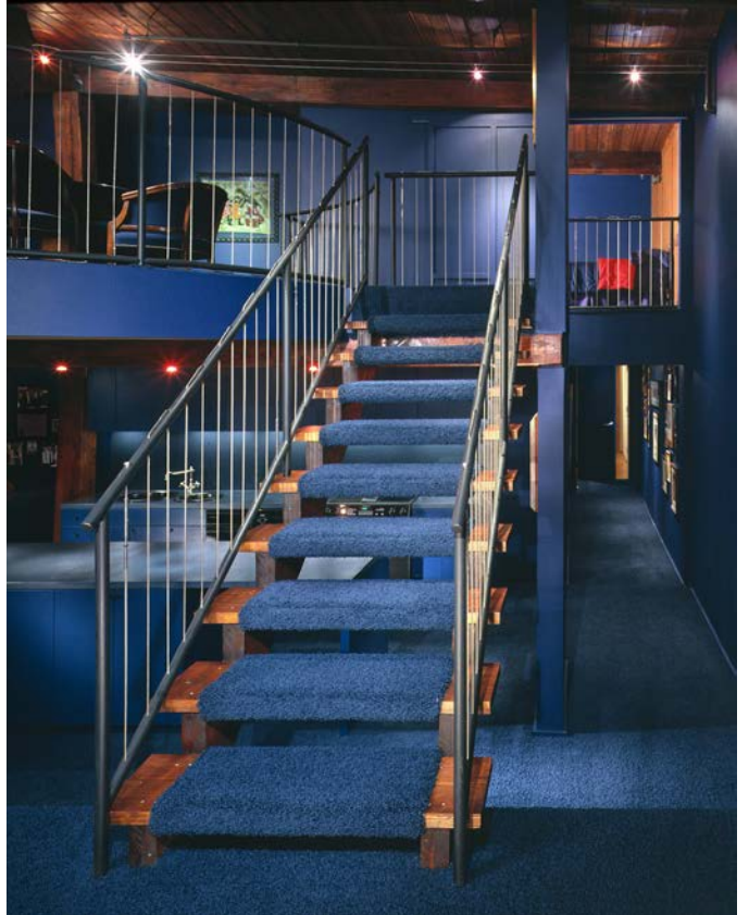
Stair to mezzanine with "woven" cable handrail. View looking east.
