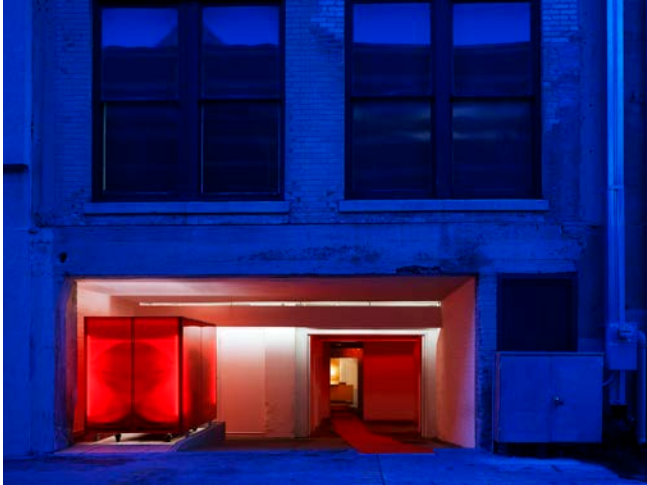
The alley entry serves as the primary delivery access for RED Prime Steak Restaurant. It is also the Ghost Gallery entrance. For events, a 100' red carpet rolls out from the alley to the gallery. A red polycarbonate box encloses the used cooking oil container.
