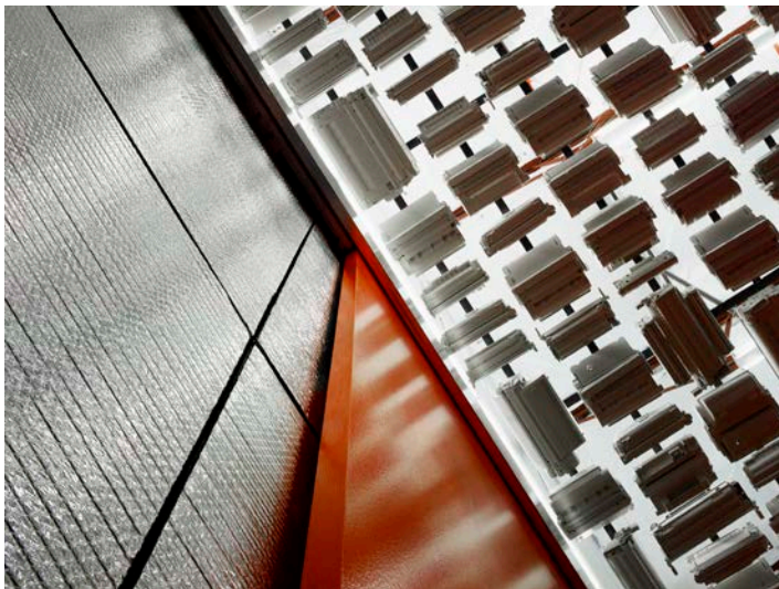
A detail of the training room ceiling and orange sliding wall panel.
