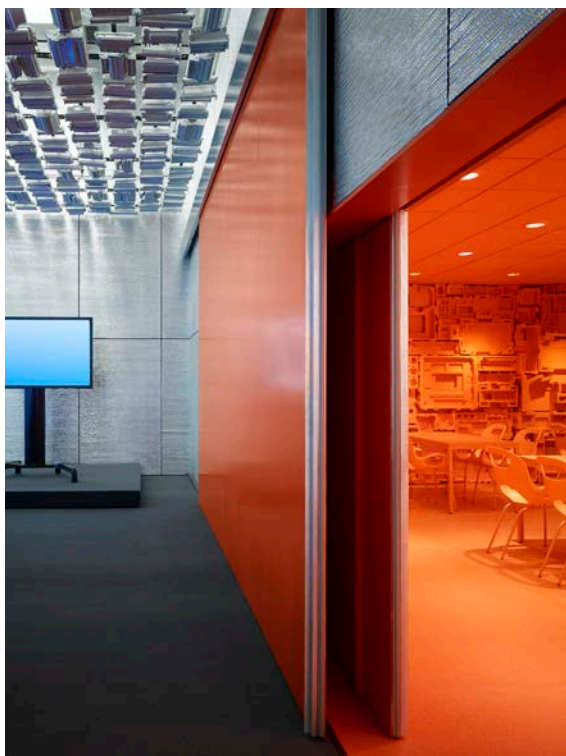
A pair of 30' wide sliding doors separates the training room from the café.
