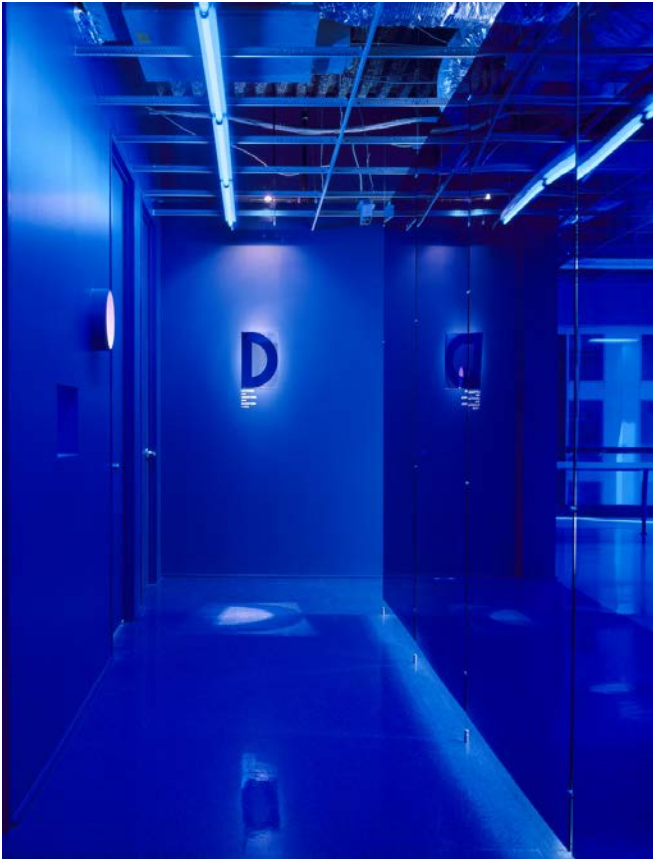
Looking west down corridor past production to find the "Big D" panel
