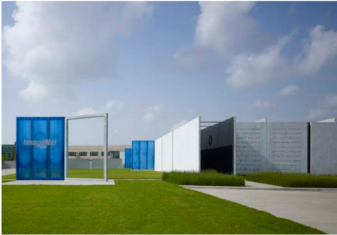
Main entry looking south
