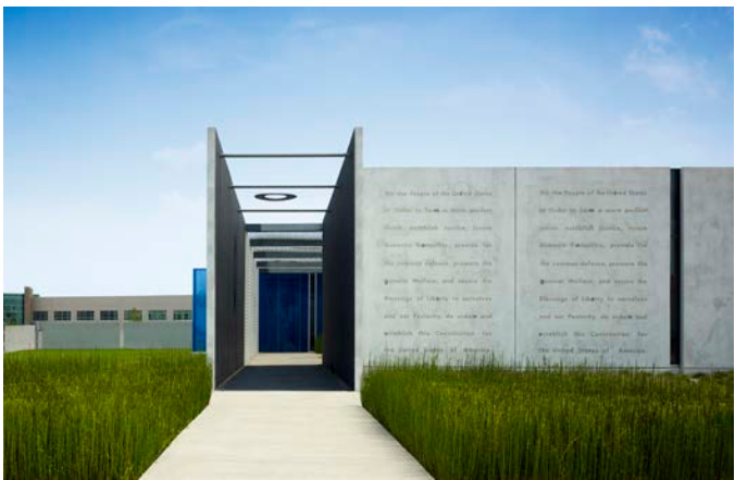
The Preamble to the Constitution is sand blasted onto the concrete panels as a duplicate, with the letters for "ImageNet" cast through the panel
