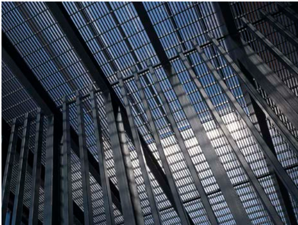
North stair detail looking up through steel grating and "stick framing."
