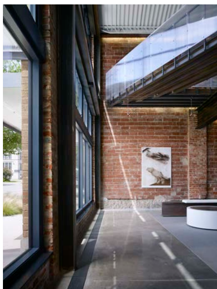
The main entry lobby showing the wide flange bracing on the south wall, the exposed masonry, and the second floor bridge.
