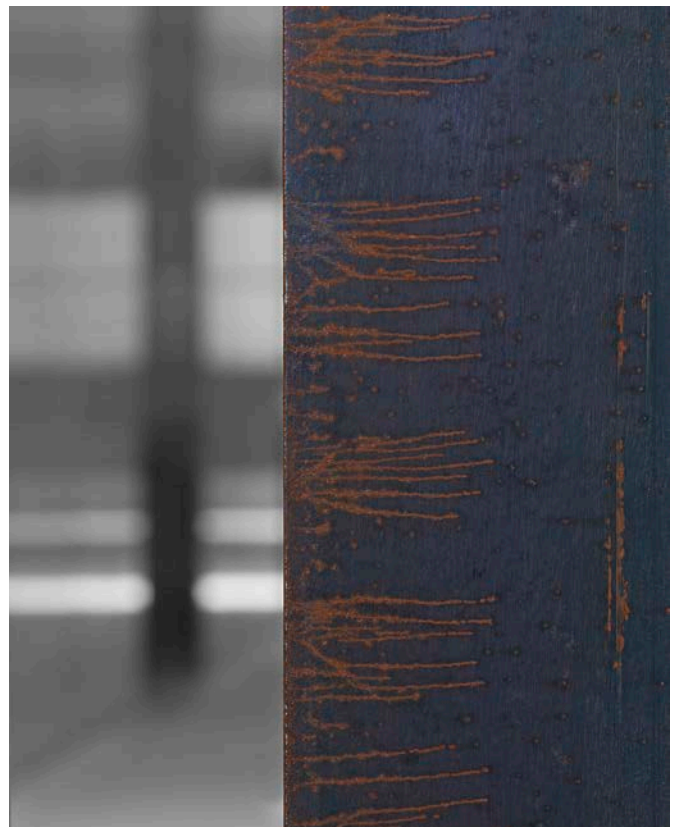
Fabrication "scars" are celebrated as art. All the steel was waxed to stop the rusting.
