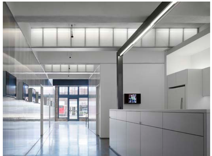
View from kitchen gallery looking south towards main entry. New polycarbonate clad beams were created to house plumbing, fire protection and electrical routing. A steel portal frame lights the main countertop.
