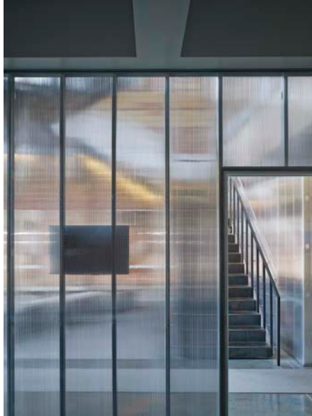
View from main conference room looking west at new folded steel stair. This image illustrates the beauty of the transparent polycarbonate and its reaction to light and surface.
