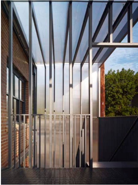
Detail of north fire stair and deck. Polycarbonate roof and wall are attached to the steel framing. This supports the idea of "stick framing."
