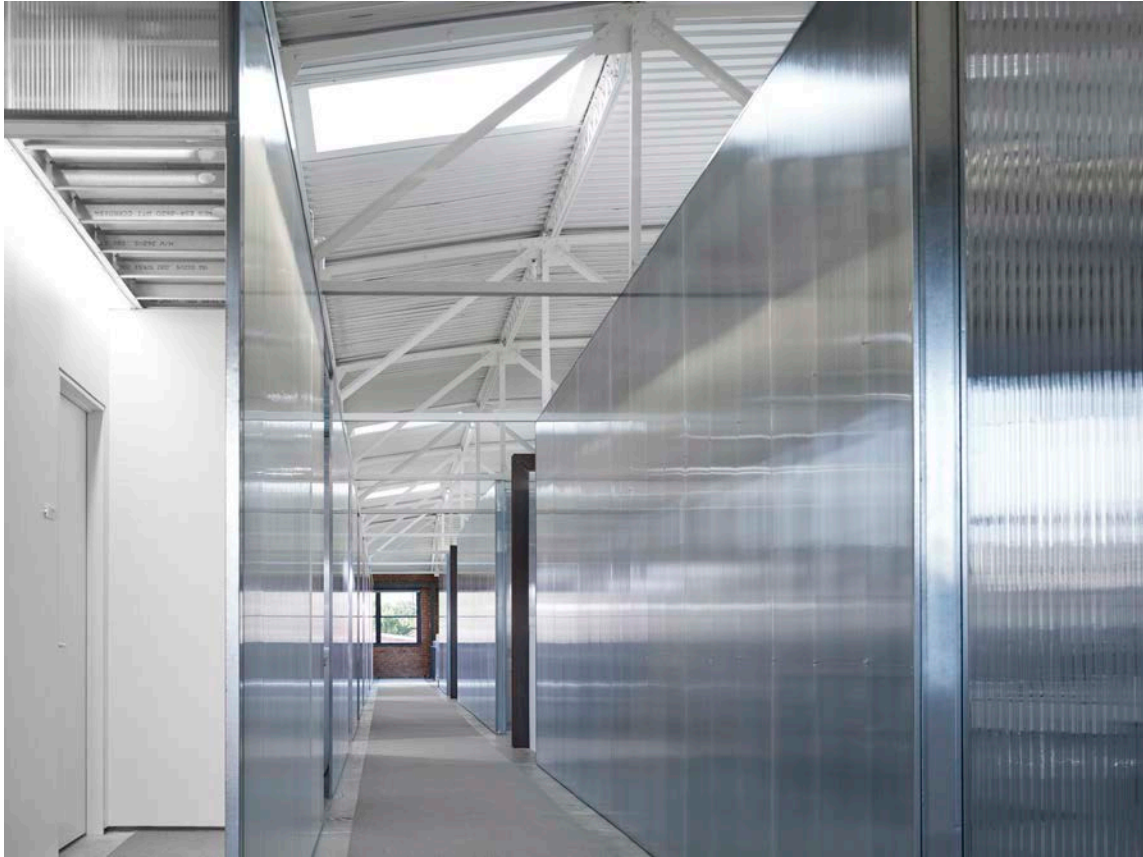
The 2nd floor workspace corridor is asymmetrically placed in order to take advantage of the existing skylight locations. The polycarbonate is transparent, reflective and private all at once.
