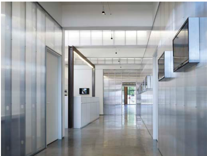
Main entry gallery with polycarbonate panels over steel studs. Project images are in a slide show on the plasma screens on the right. The steel portal defines the serving kitchen. The original beam structure remains and we added a lighted translucent duplicate to house lighting, fire protection and HVAC.
