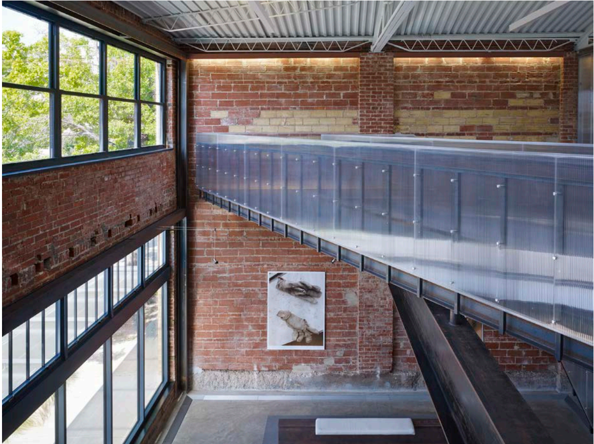
The entry lobby overlook showing historic beam pockets on the left, the 1930s bowstring truss roof, and the new steel and polycarbonate bridge.
