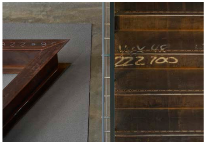
Detail of folder steel stair showing the fabrication marks left in place. All of the steel is waxed to protect from rusting. A custom nosing was created to make the stair treads non slip.
