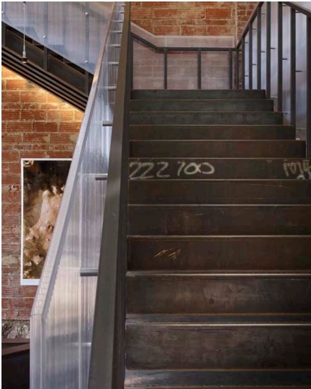
Ground floor stair landing view of the folded steel stair and shop markings.
