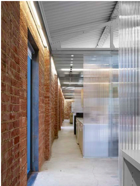
West service corridor that places all of the office equipment adjacent to the project manager workspaces. Intentionally masonry was left exposed and the new millwork adjacent to it.
