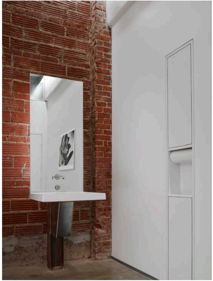
Typical toilet lavatory detail showing freestanding pedestal sink clad in steel panels. A light behind the mirror accentuates the clay tile texture. On the right is a custom made towel holder and trash dispenser.
