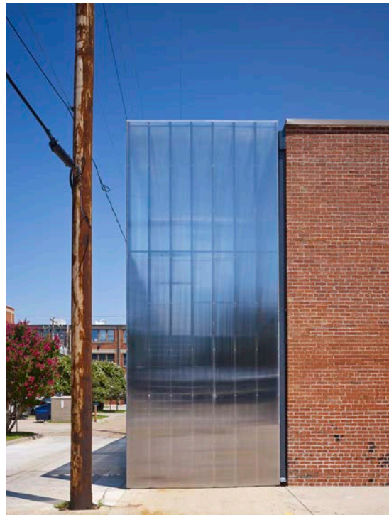
This is the northwest corner showing the polycarbonate addition on the north side. We embraced the alley aesthetic.
