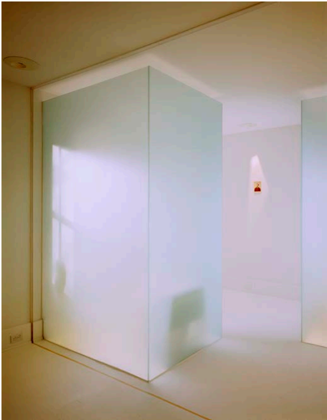
View looking southwest at water closet "light vessel"
