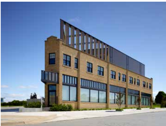
South elevation illustrating the 3rd floor glass addition and the protected outdoor deck. Triangular shaped down spouts show consistent detailing.
