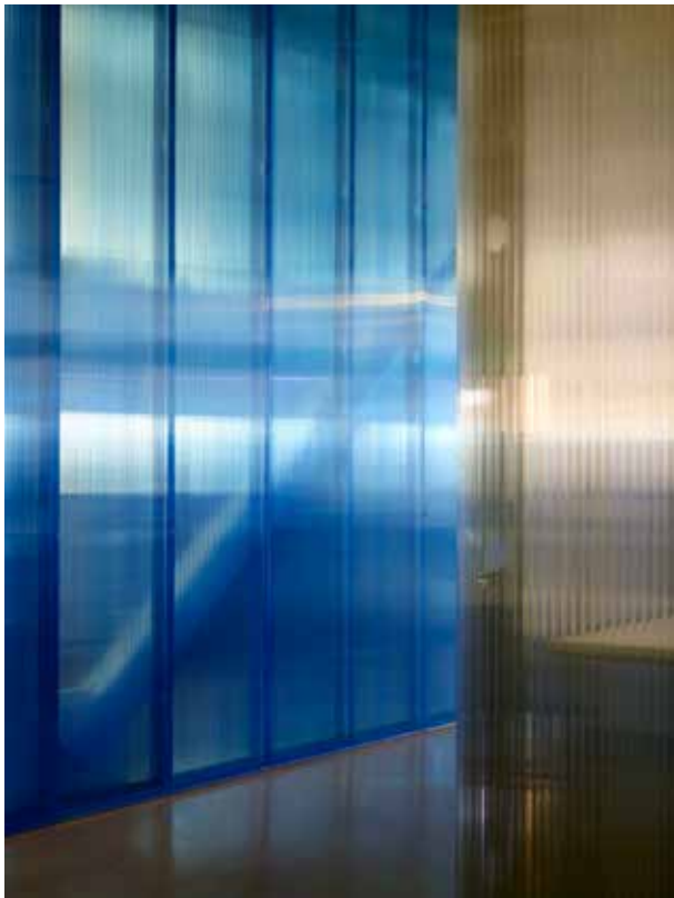
Polycarbonate panels provide acoustical and visual privacy and give exposed structure a ghostly quality.
