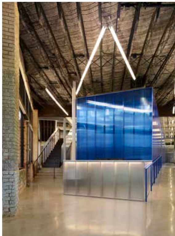
View from the flatiron entry towards the reception desk. The blue polycarbonate office core defines new vs. historic. The original exposed metal lath and concrete deck above remains. Floors are polished concrete.
