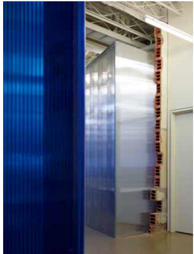
The existing clay tile firewall at the historic stair remains in place.
