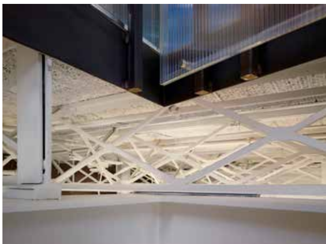
A journey using the ceremonial stair shows exposed historic flat steel structural joists
