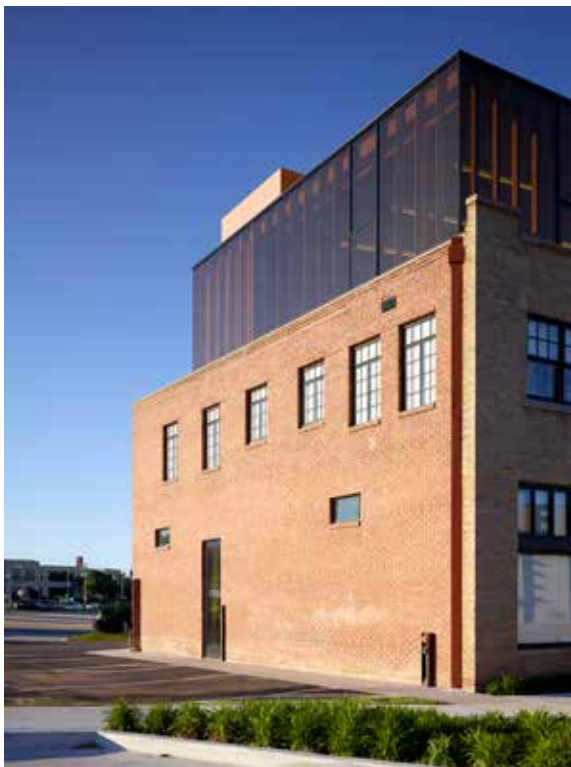
The east elevation illustrates the historic “back” of the building. Previously filled-in windows are reopened and the common red brick was cleaned. The 3rd floor addition sets back away from the parapet in respect.
