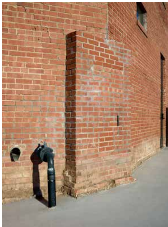
Original incinerator access was filled-in in the 1960s. The existing form remains with the original exposed steel door pull.
