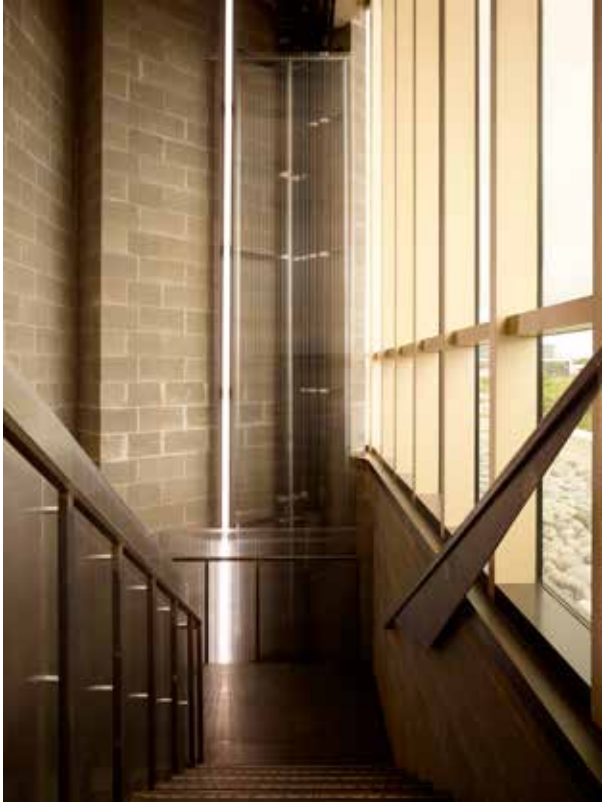
The east fire stair celebrates exposed vertical piping with a folded steel plate stair and large 3 rd floor glass.
