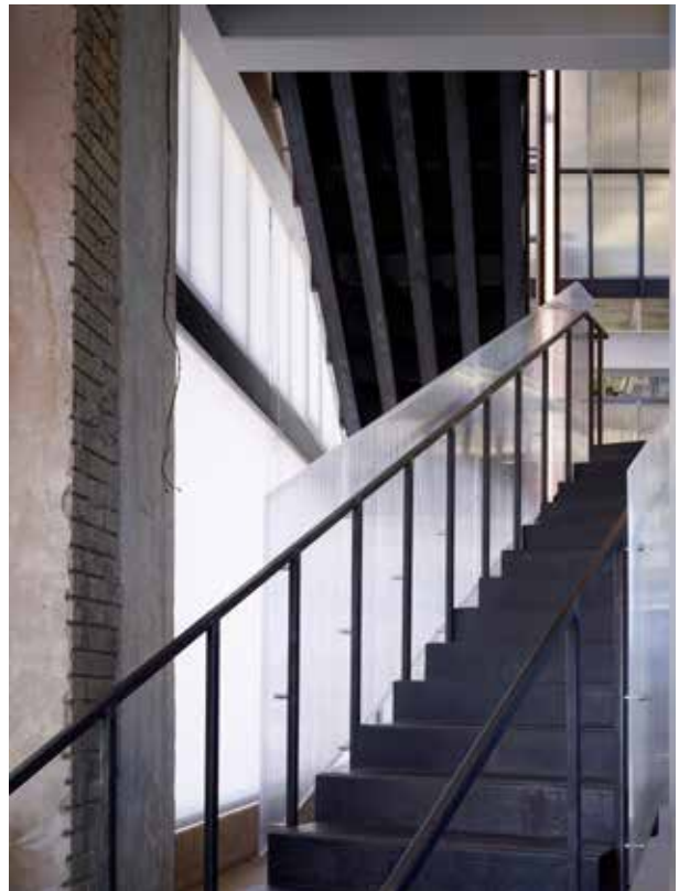
The ceremonial stair shows folding steel plate, risers and treads, and 1" square solid stock pickets.
