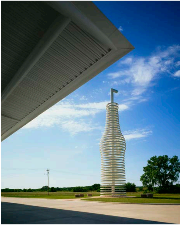
Canopy/Bottle detail looking northwest
