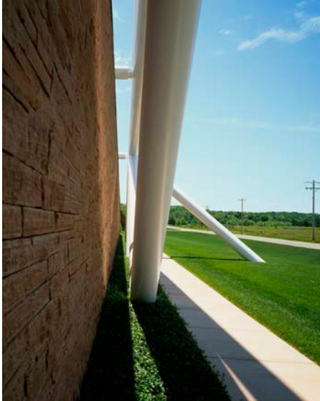
View along west stone wall looking south showing stone wall/structure detail.
