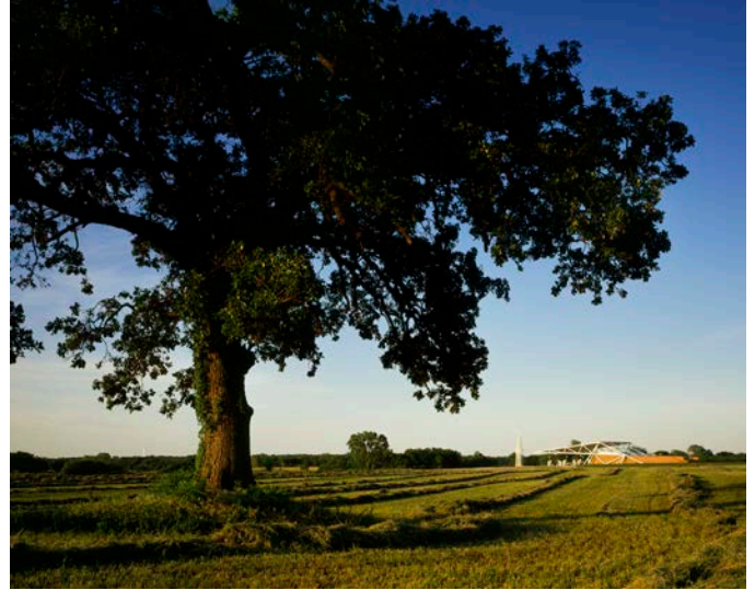
West elevation from adjacent field
