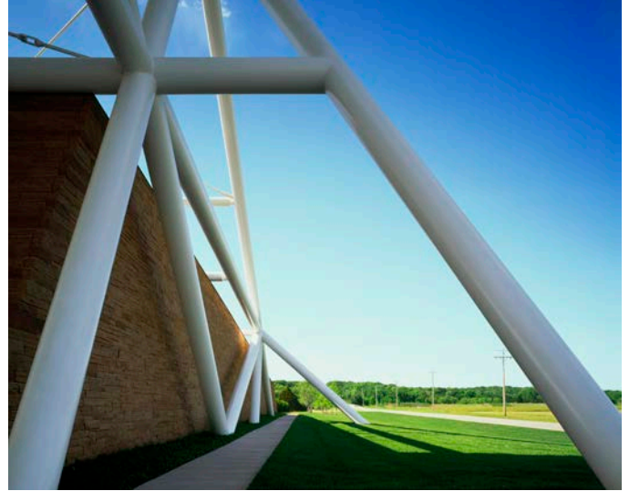
West elevation stone wall/structure detail
