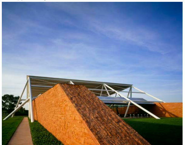
Southwest corner of stone wall/courtyard
