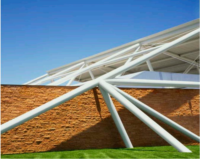
East elevation with stone wall and structure detail
