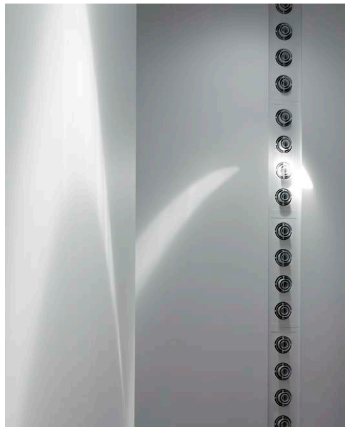
Skylight reflection and nozzle detail
