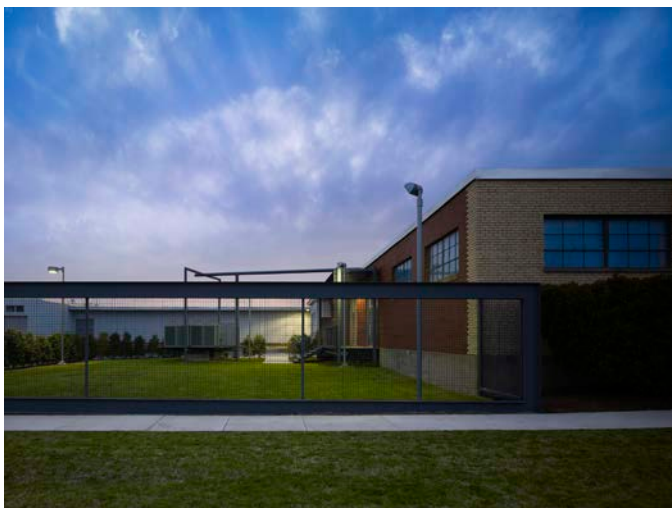
Equipment courtyard with picture window portal looking west
