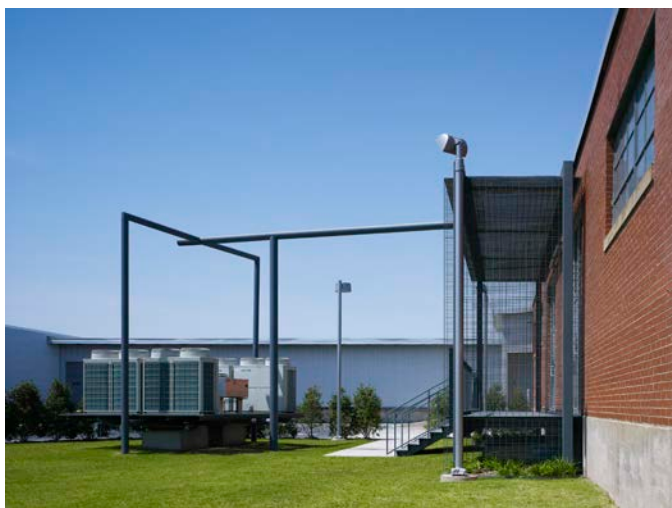
Equipment courtyard looking west
