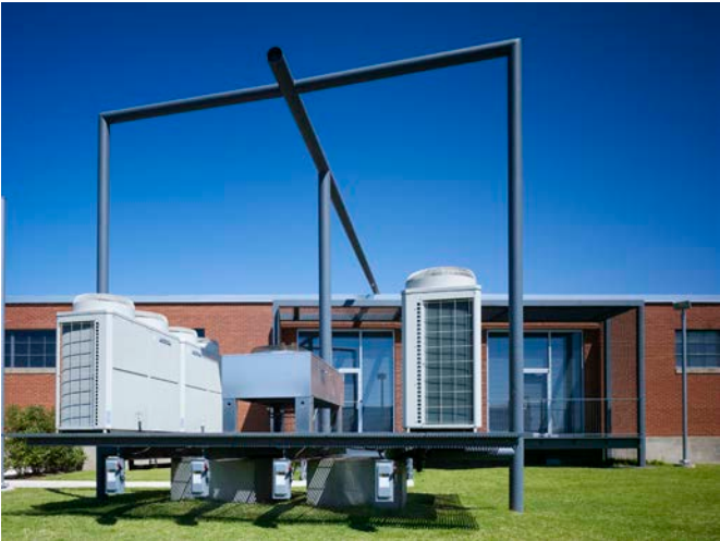
Equipment courtyard looking north
