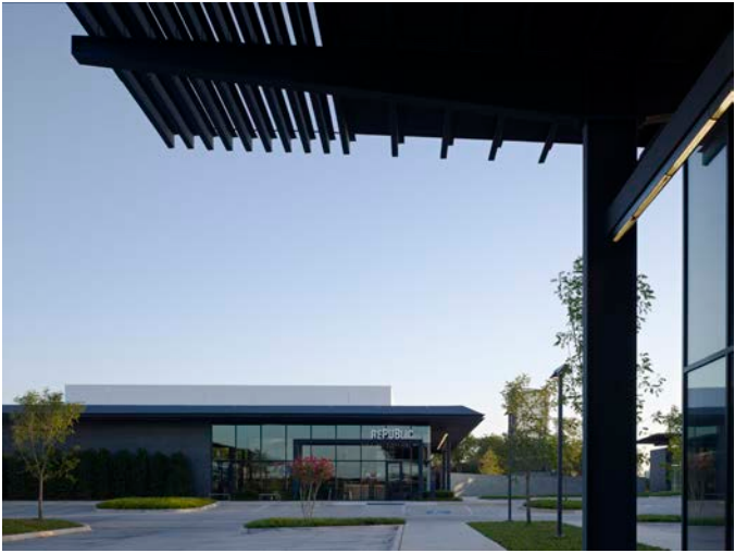
South elevation from adjacent retail building
