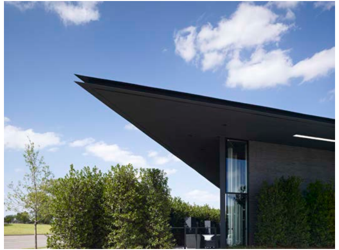
Southwest corner of building with hedge wall patio enclosure
