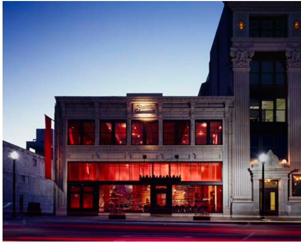
Main Entry/West elevation
