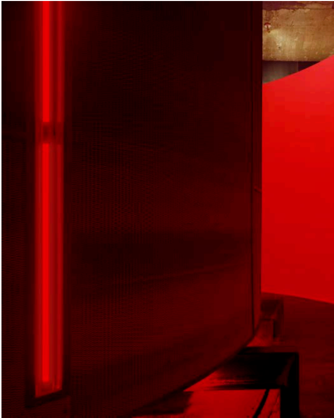
Turntable detail showing metal mesh steel structure and historic steel turntable
