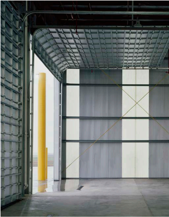
Southeast corner of equipment storage area
