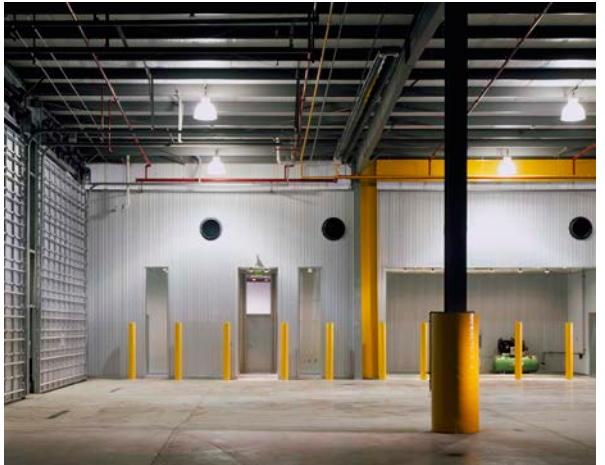
Looking north from equipment storage area towards offices and tire change
