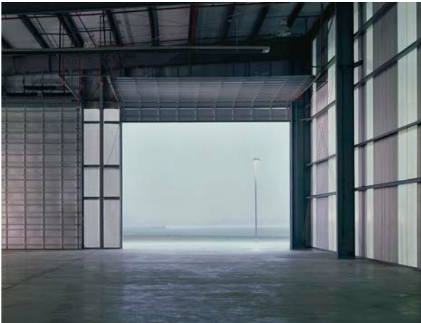
Southeast corner service door
