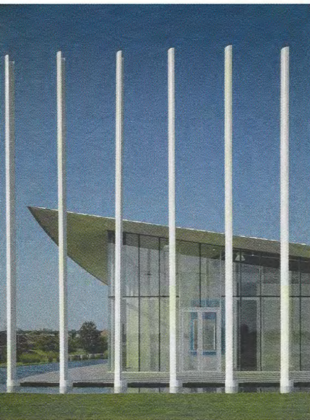
The lobby of the boathouse (top). Elliott and project architect Brian Fitzsimmons stained the structural concrete slab to serve as an all-purpose floor, and the reception desk is encased in blue Plexiglas and translucent polycarbonate. The faceted steel pylons at the entrance (above) withstand the strong winds that sweep across the prairie.
